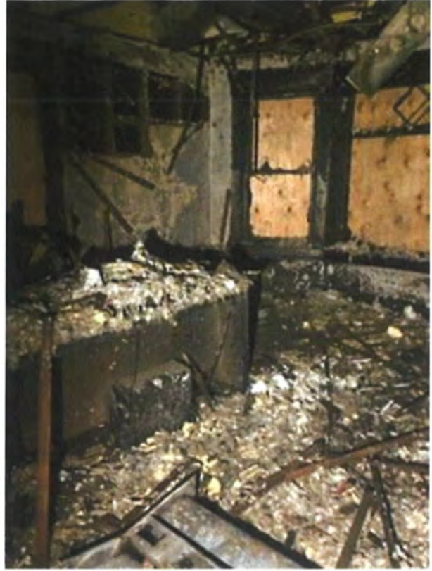
Photo 8. Office with bay window (2024).
