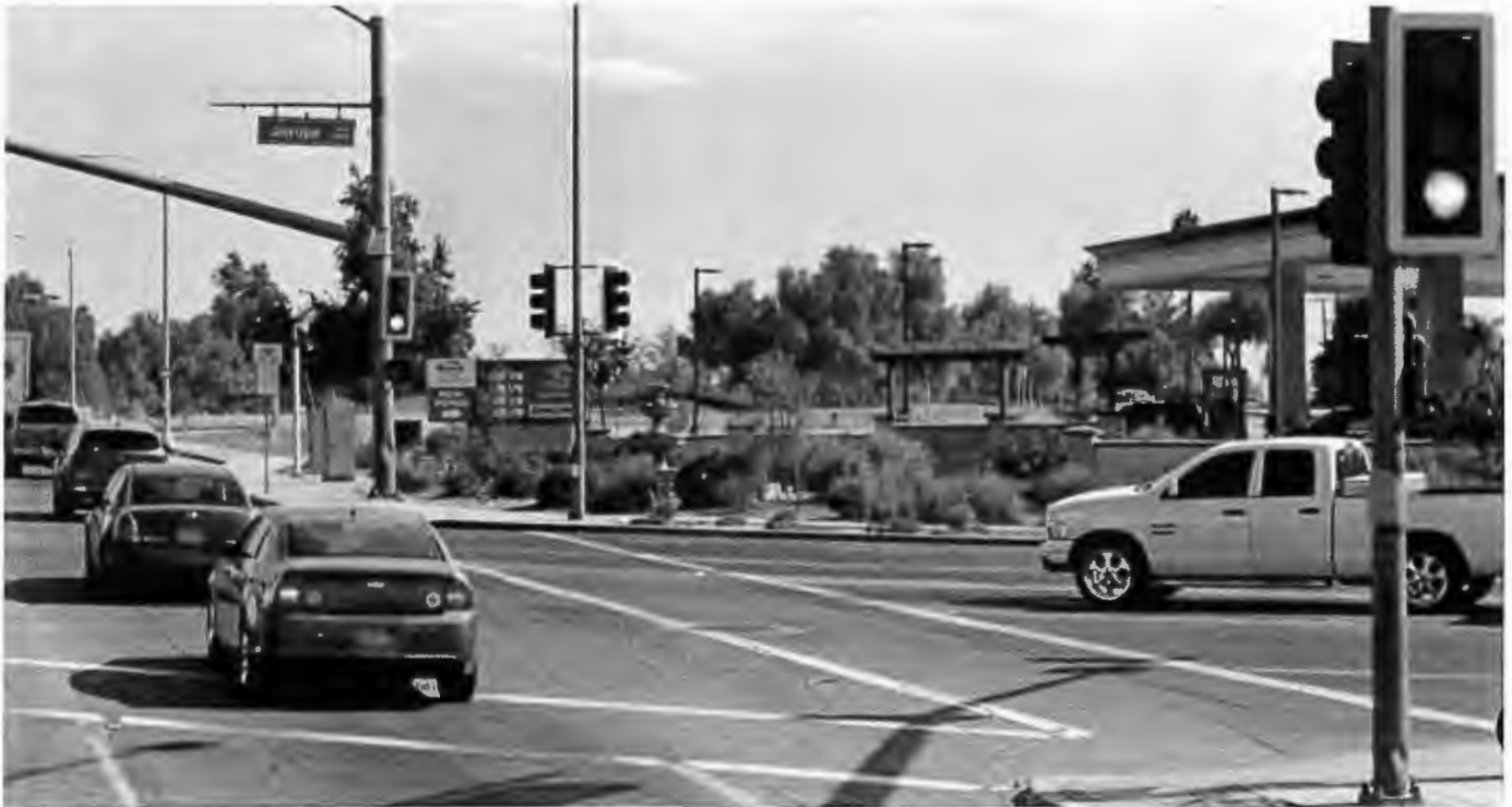
Intersection 12 – Van Buren Blvd & Jurupa Ave - Looking southbound. Improvements include – high visibility crosswalks, green bike lane striping & audible pedestrian pushbuttons.
