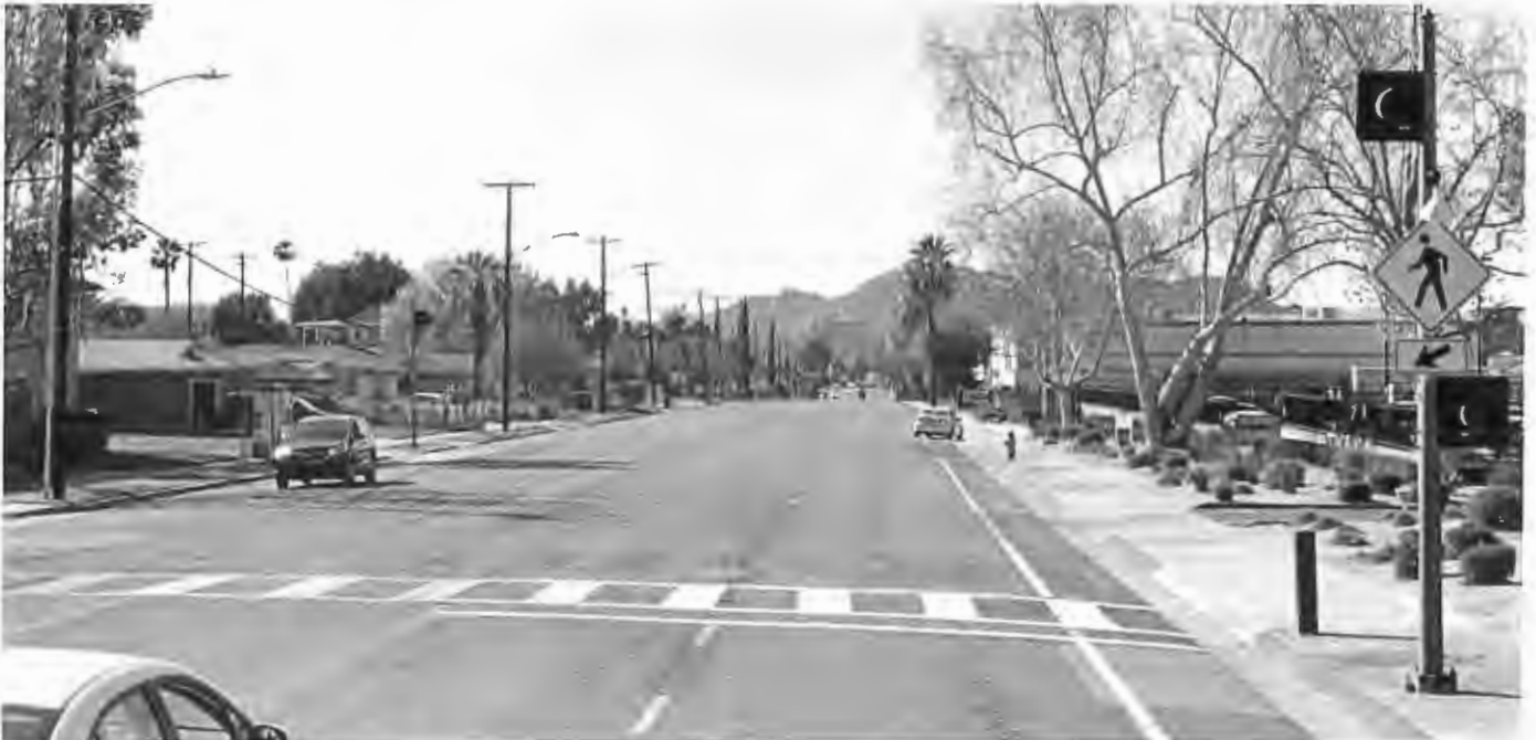
Intersection 6 – Third St & Anderson Ave - Looking westbound. Improvements include – rectangular rapid flashing beacon
