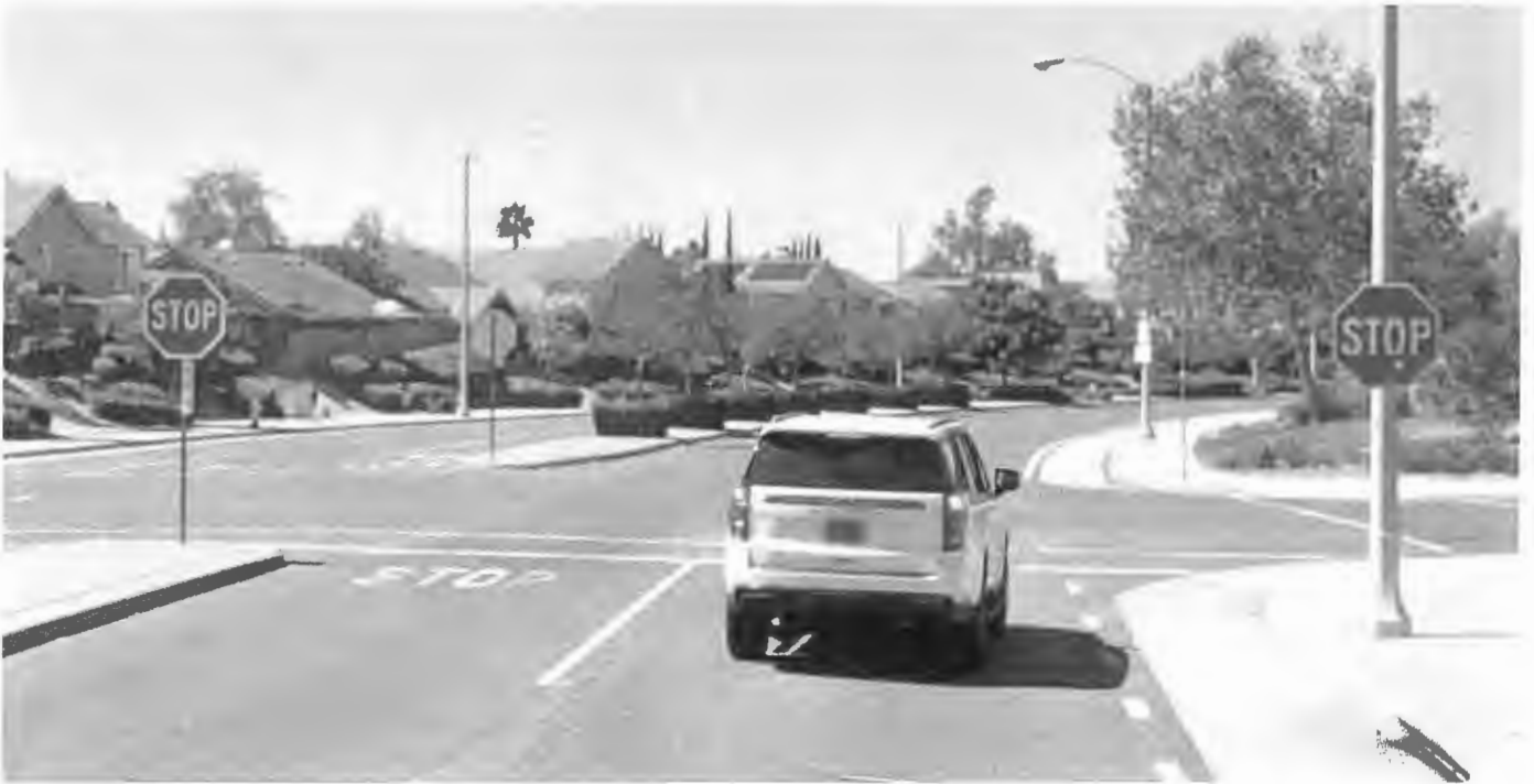
Intersection 9 – Orange Terrace Pkwy & Abrams Dr - Looking westbound. Improvements include – high visibility crosswalks & flashing LED-edge lit stop signs. (Top picture)
