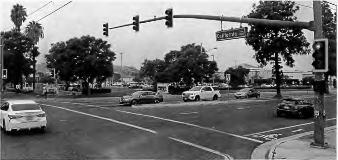
Intersection 15 – Van Buren Blvd & California Ave - Looking northbound. Improvements include – high visibility crosswalks & audible pedestrian pushbuttons. (Top picture)
