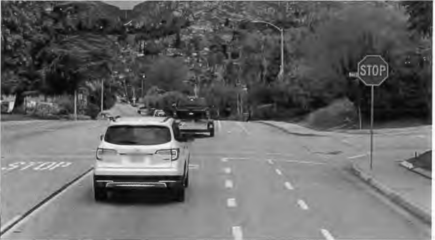
Intersection 5 – Watkins Dr & Knox Ct - Looking northbound. Improvements include – high visibility crosswalk & flashing LED edge-lit stop signs. (Top picture)
