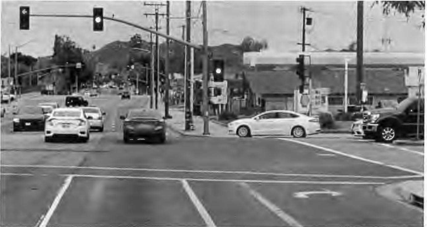
Intersection 1 - Blaine St at Iowa Ave - Looking westbound. Improvements include – high visibility crosswalk, green bike lane striping & audible ped push buttons. (Top picture)
