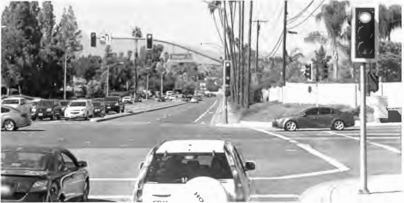
Intersection 7 – Alessandro Blvd & Chicago Ave - Looking northbound. Improvements include – high visibility crosswalk, green bike lane striping & audible pedestrian pushbuttons. (Top picture)
