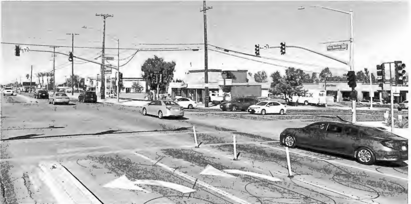
Intersection 11 – Wood Rd & Van Buren Blvd - Looking westbound. Improvements include – high visibility crosswalks, green bike lane striping & audible pedestrian pushbuttons. (Top picture)
