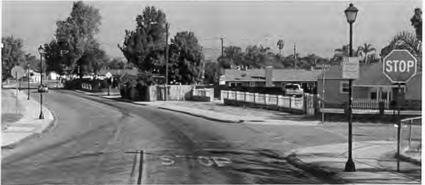
Intersection 17 – Rutland Ave & Sylvan Dr - Looking northbound. Improvements include – high visibility crosswalks & flashing LED-edge lit stop signs. (Top picture)
