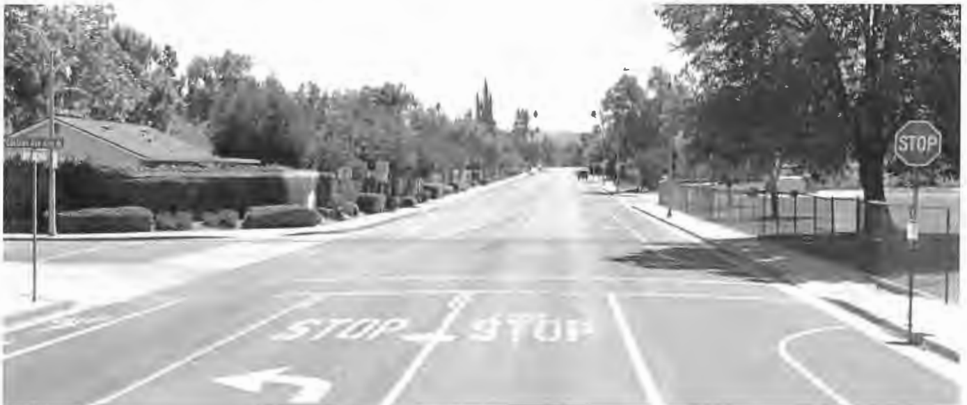
Intersection 22 – Golden Ave & Cochran Ave - Looking southbound. Improvements include – high visibility crosswalks & flashing LED-edge lit stop signs.
