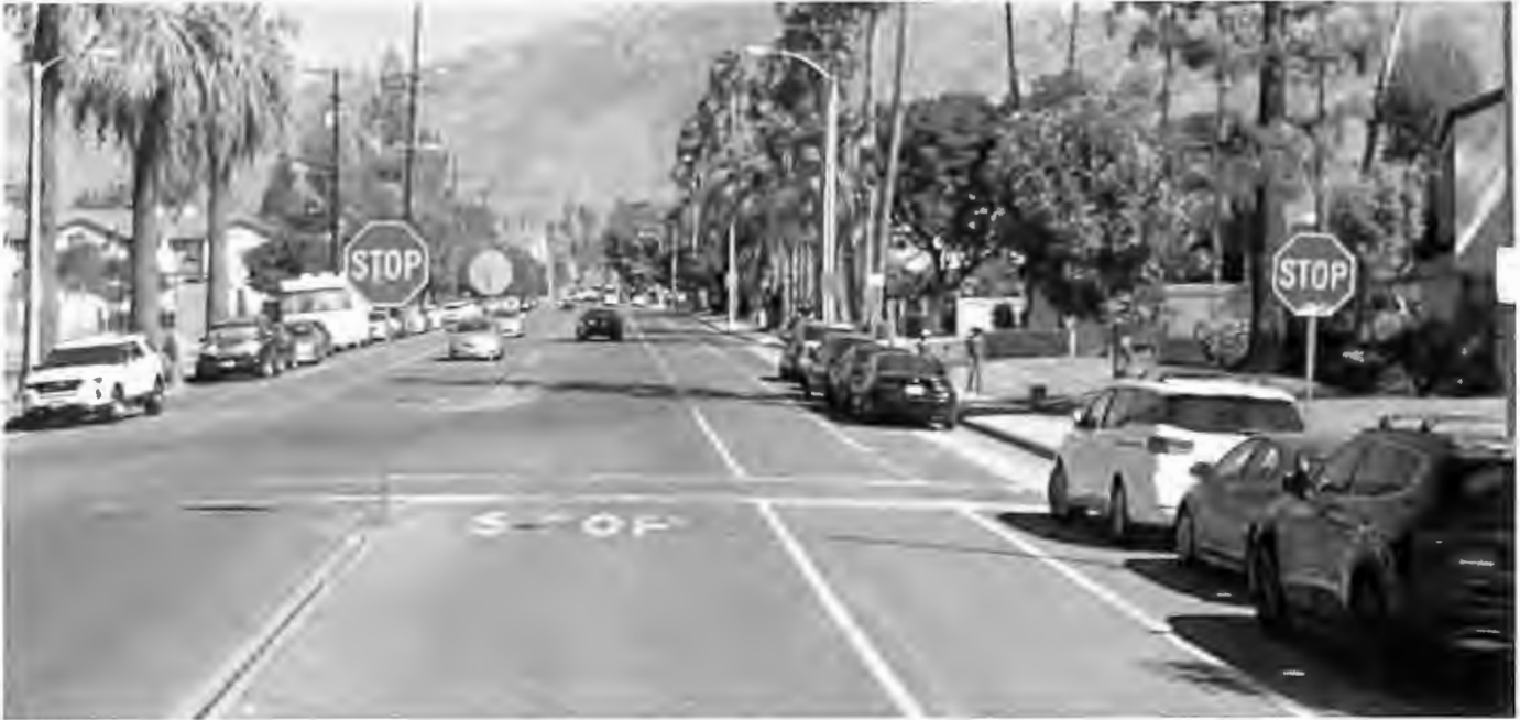
Intersection 3 – Rustin Ave & Linden St - Looking eastbound. Improvements include – high visibility crosswalk, green bike lane striping & flashing LED edge-lit stop signs. (Top picture)
