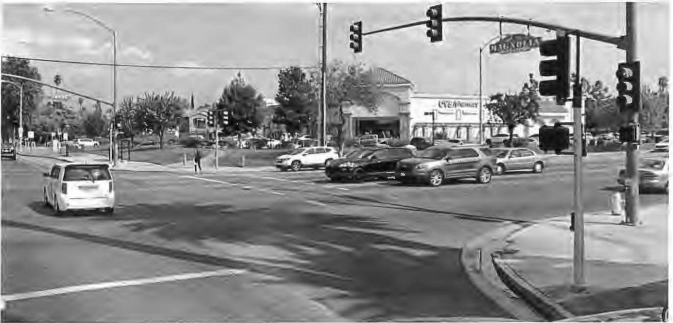
Intersection 14 – Adams St & Magnolia Ave - Looking eastbound. Improvements include – high visibility crosswalks, green bike lane striping & audible pedestrian pushbuttons.
