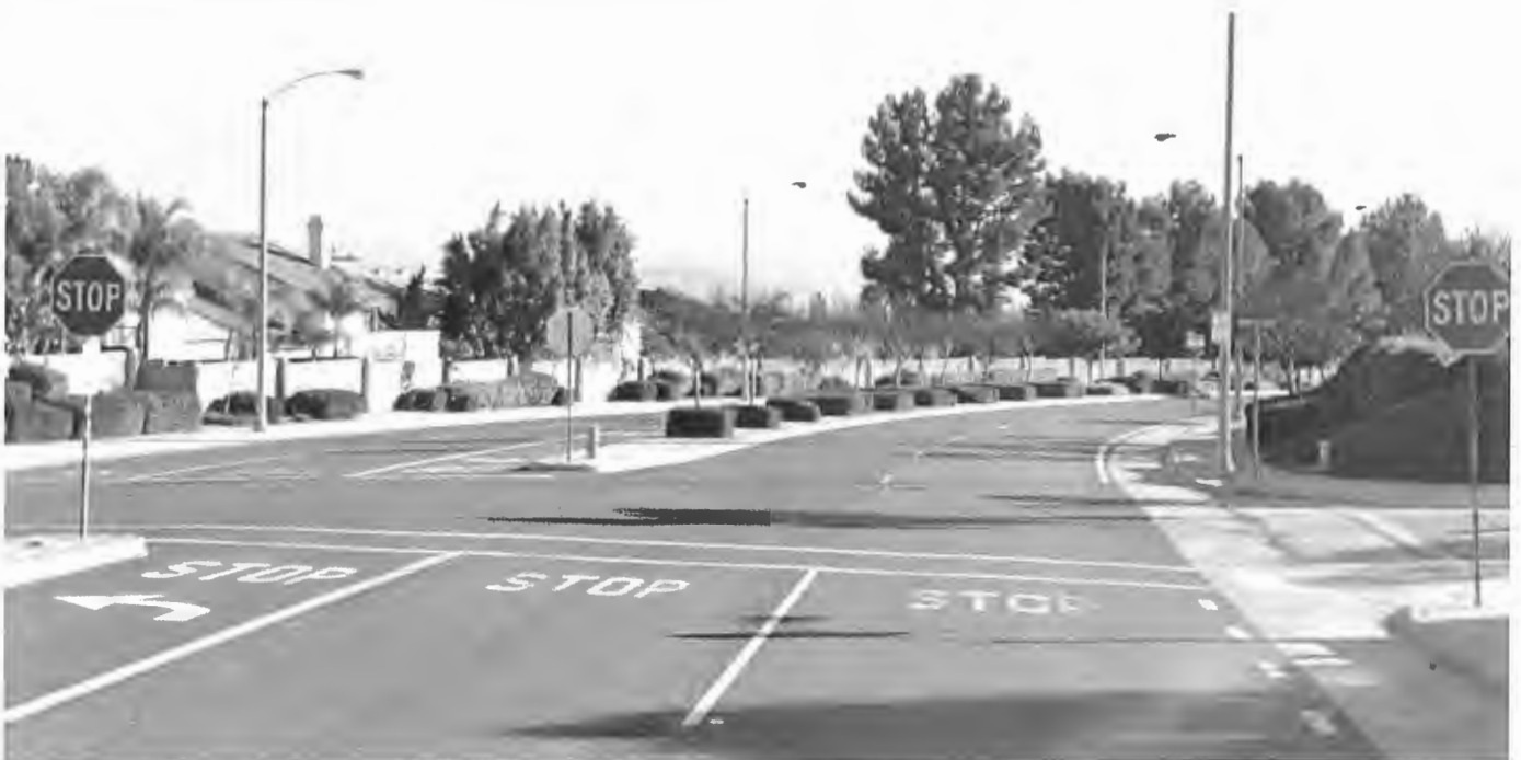
Intersection 10 – Orange Terrace Pkwy & Sandhill Dr. (west)- Looking eastbound. Improvements include – high visibility crosswalks & flashing LED-edge lit stop signs.
