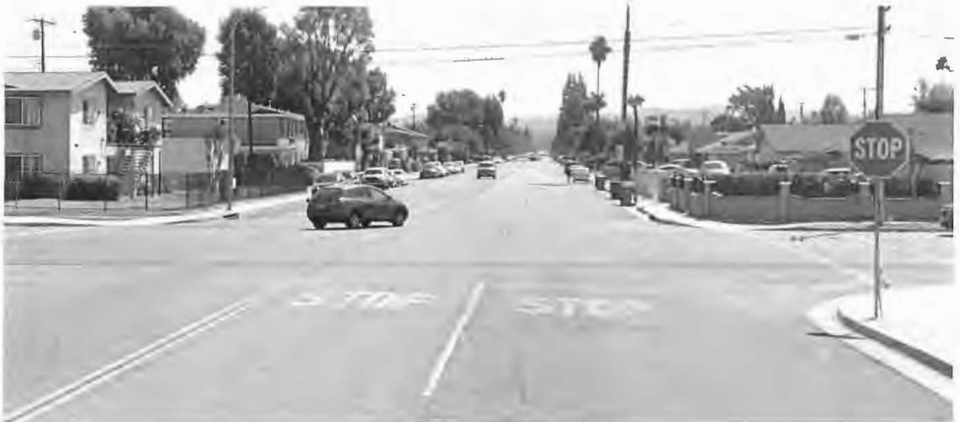
Intersection 18 – Collett Ave & Polk St - Looking southbound. Improvements include – high visibility crosswalks & flashing LED-edge lit stop signs.
