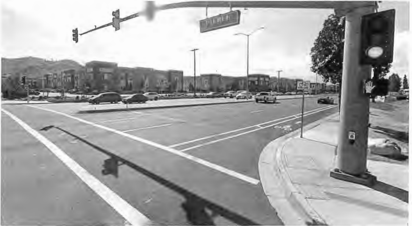
Intersection 21 – Magnolia Ave & Pierce St - Looking northbound. Improvements include – high visibility crosswalks & audible pedestrian pushbuttons. (Top picture)
