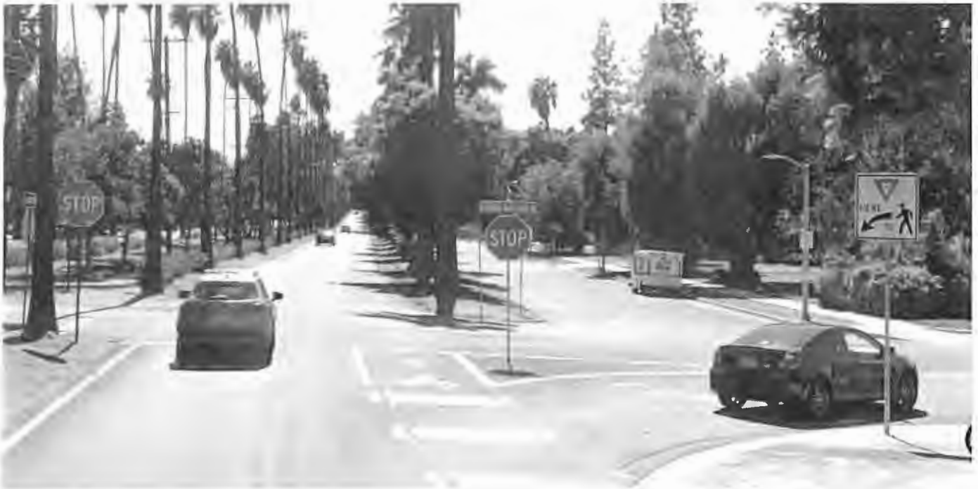
Intersection 8 – Lincoln Ave & Victoria Ave - Looking southbound. Improvements include – high visibility crosswalks, raised median & flashing LED edge-lit stop signs and pedestrian signs.
