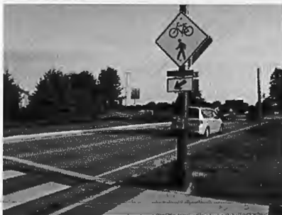
RRFBs used at a trail crossing. Source: LJB
