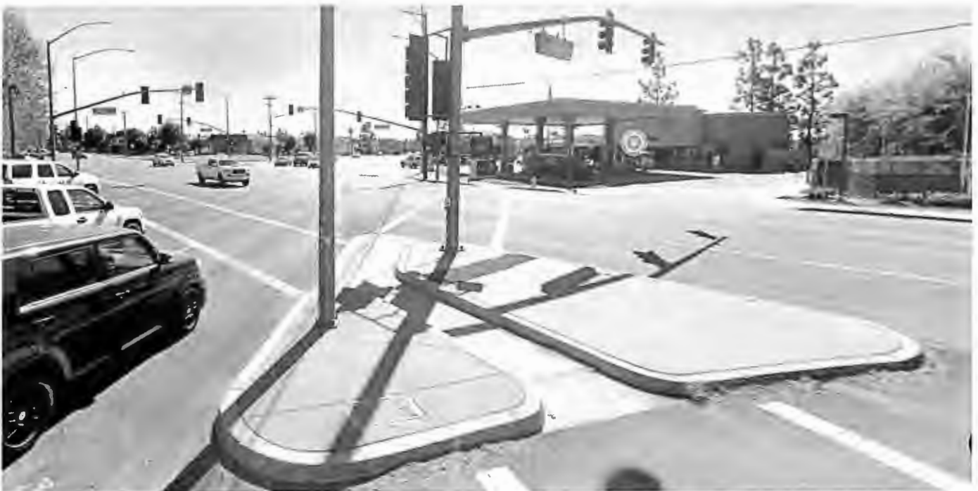
Intersection 20 – Tyler St & Hole Ave - Looking southeast. Improvements include – high visibility crosswalks & audible pedestrian pushbuttons. Note median refuge islands at two corners.
