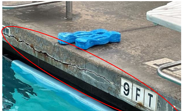
Shamel Park Pool Deck Repairs and Shade Shelter
