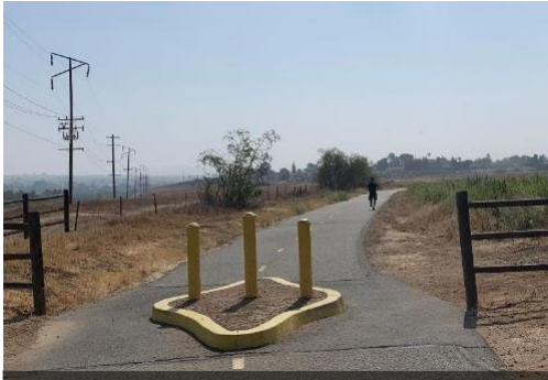
Install barriers to prevent uncontrolled access
