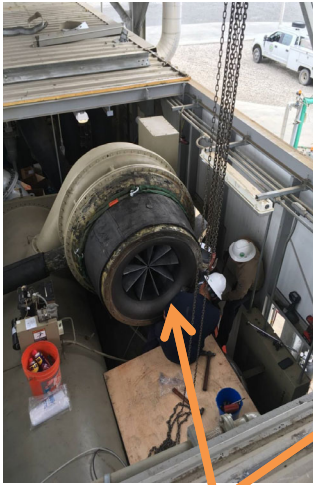
Damaged Impeller
