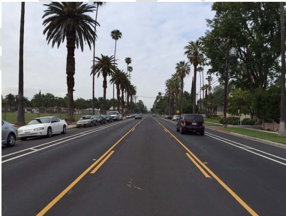
Figure 3 – 'After' Implemented 3-Lane Brockton Ave Configuration
