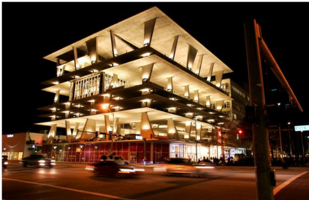
Miami Lincoln Parking Structure in Miami, Florida
