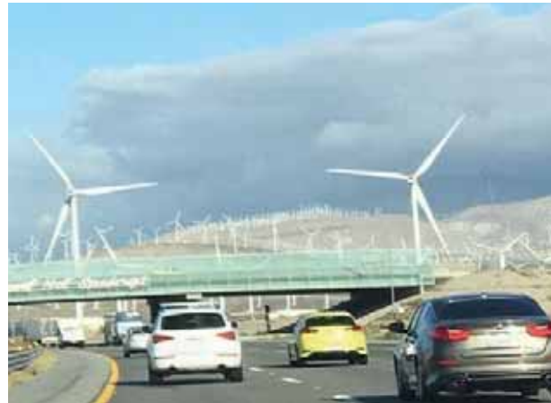
Wind turbines near the San Geronio Pass
