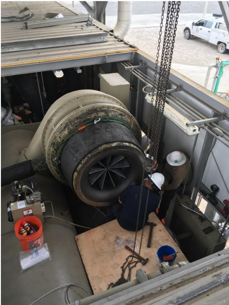
Damaged Impeller
