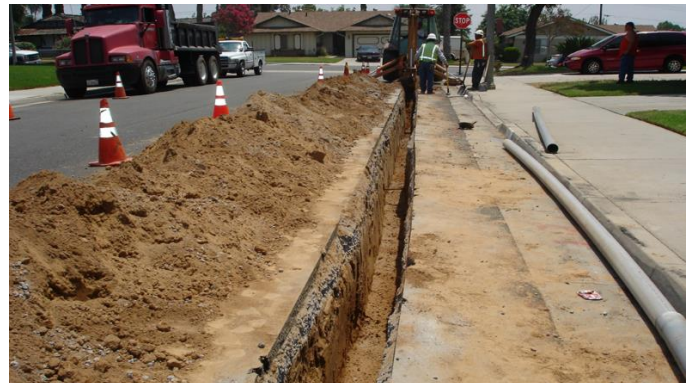
Trench and Conduit Installations
