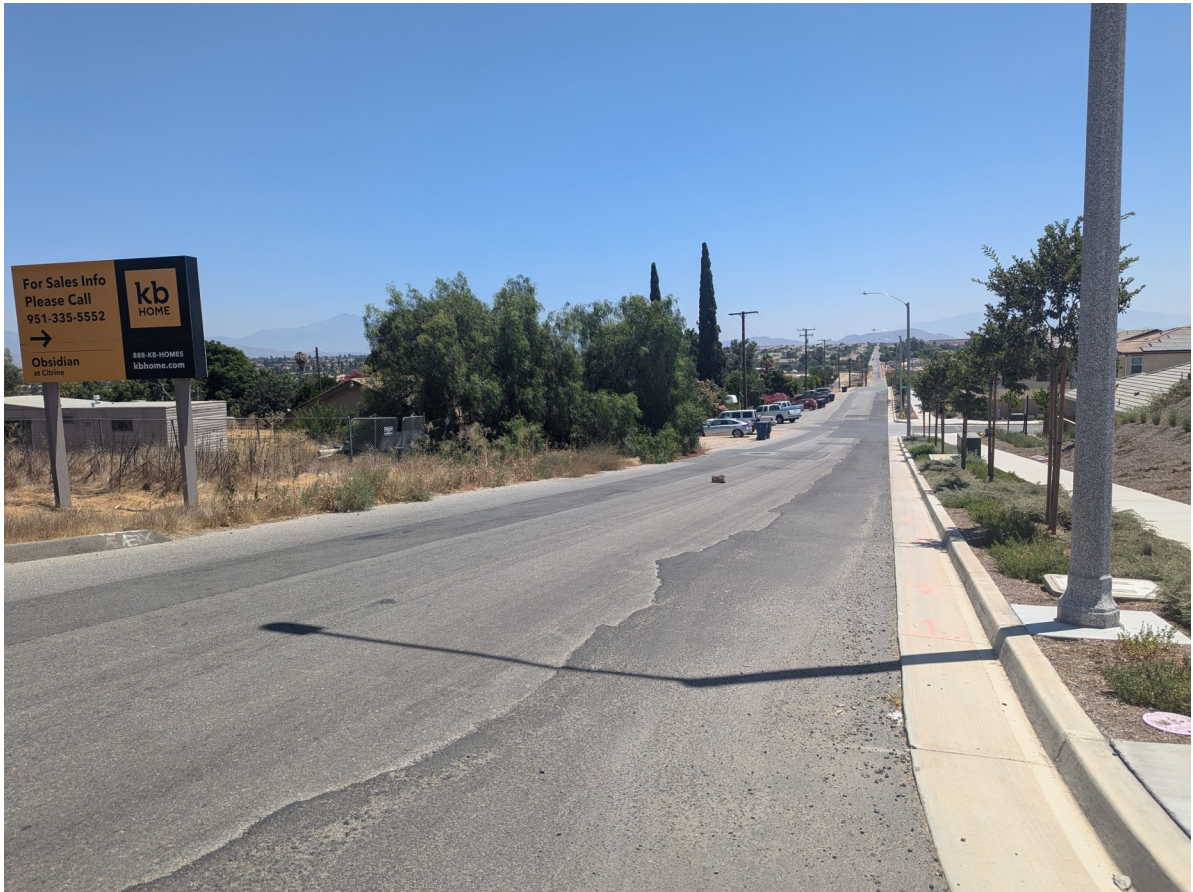
View looking east on Lurin Avenue
