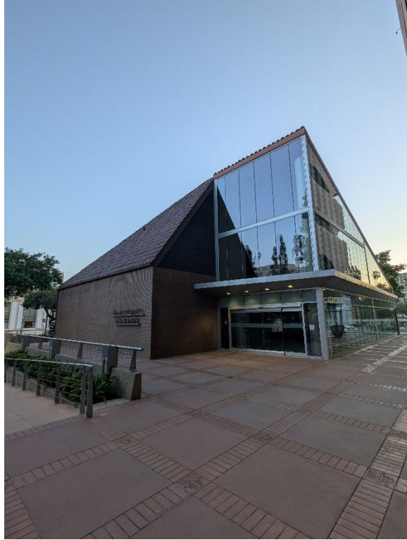
Figure 5 - Council Chambers, view looking southwest
