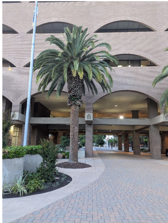
Figure 2 - Breezeway, view looking north
