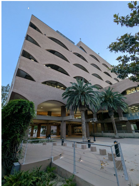
Figure 4 - North Elevation, view looking southwest
