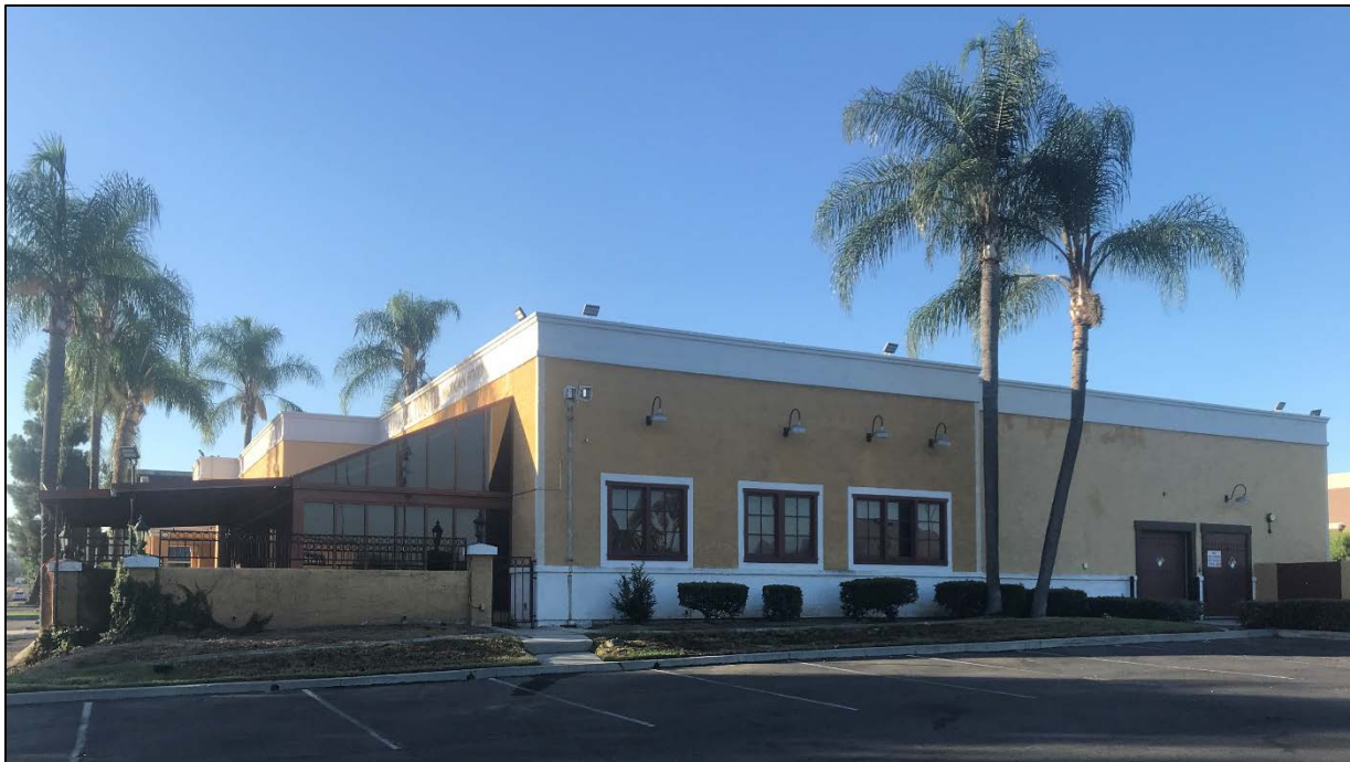
Looking south at the project site.
