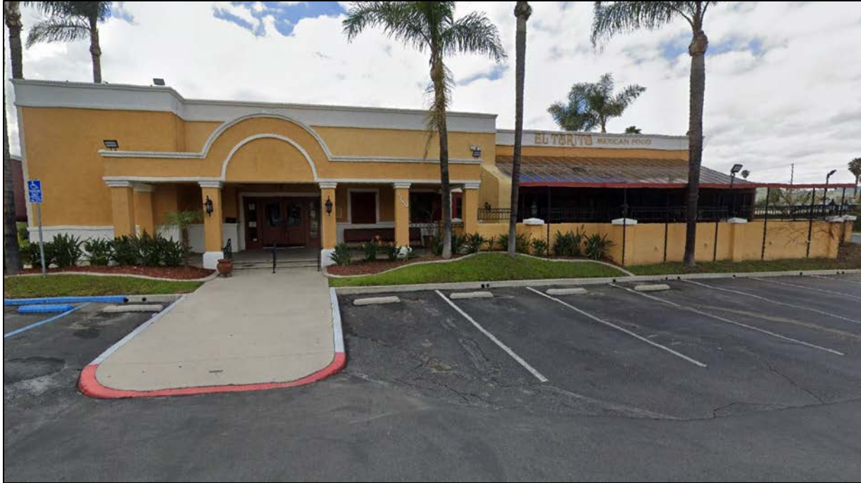
Looking west at the project site.
