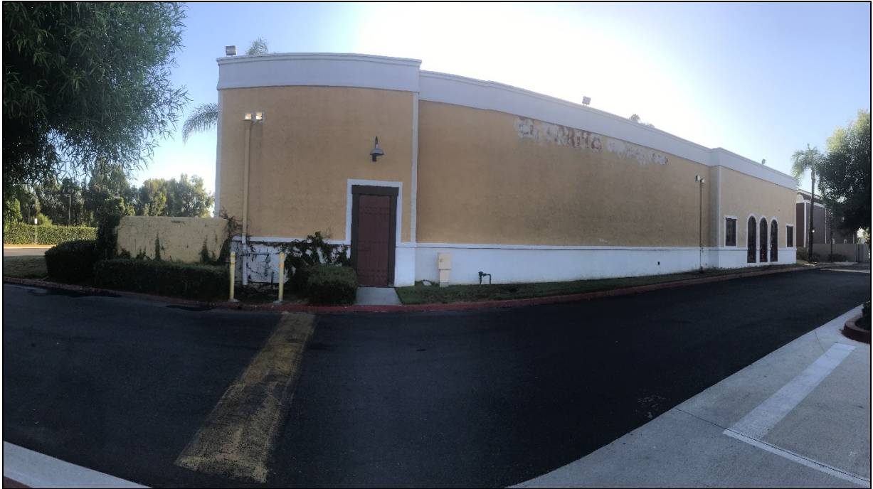
Looking east at the project site.
