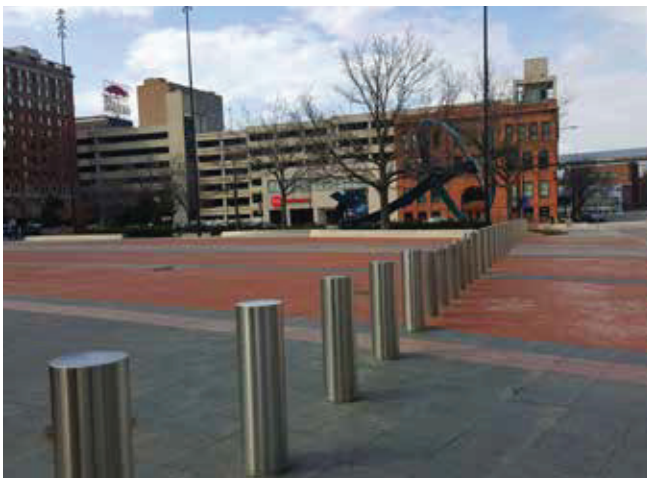
Teaming partner KPFF’s Protective Design Group provided perimeter security consulting services for the Des Moines, IA Performing Arts Center, located in the heart of downtown, on a city block with multiple entrances.
