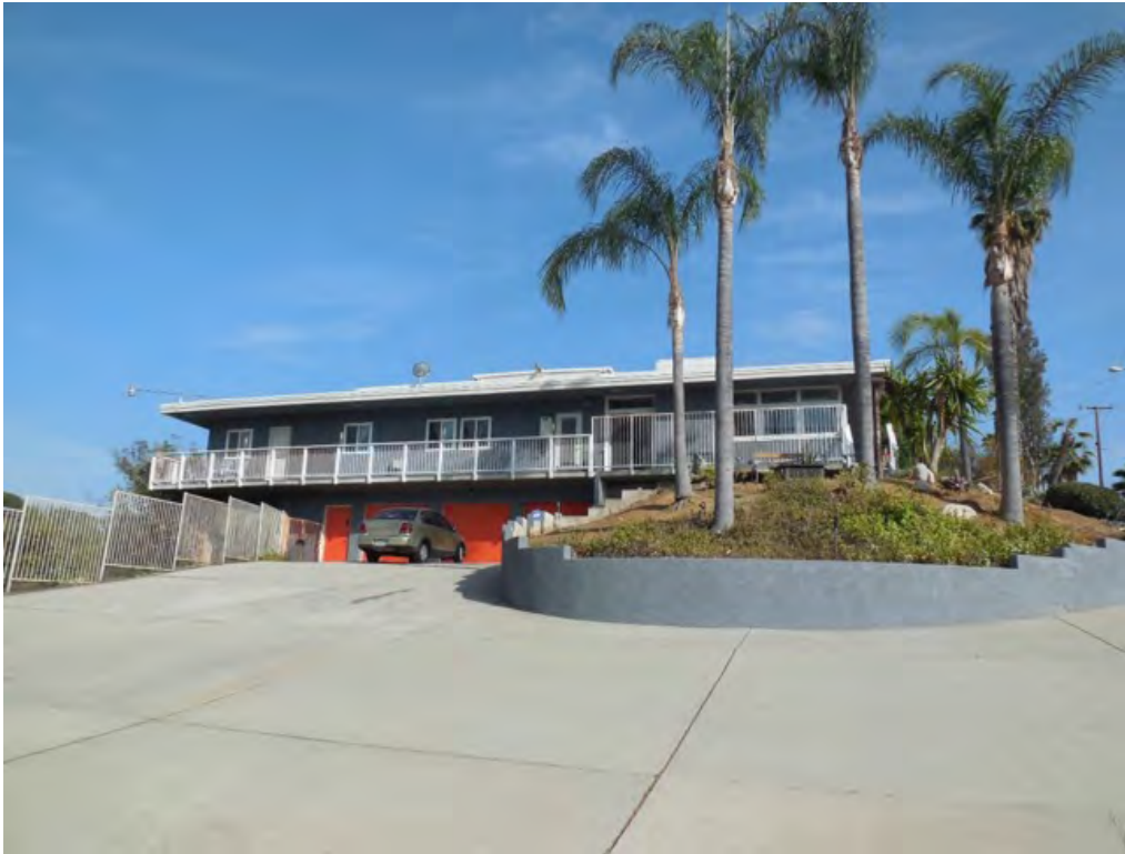
North Elevation, view looking southeast
