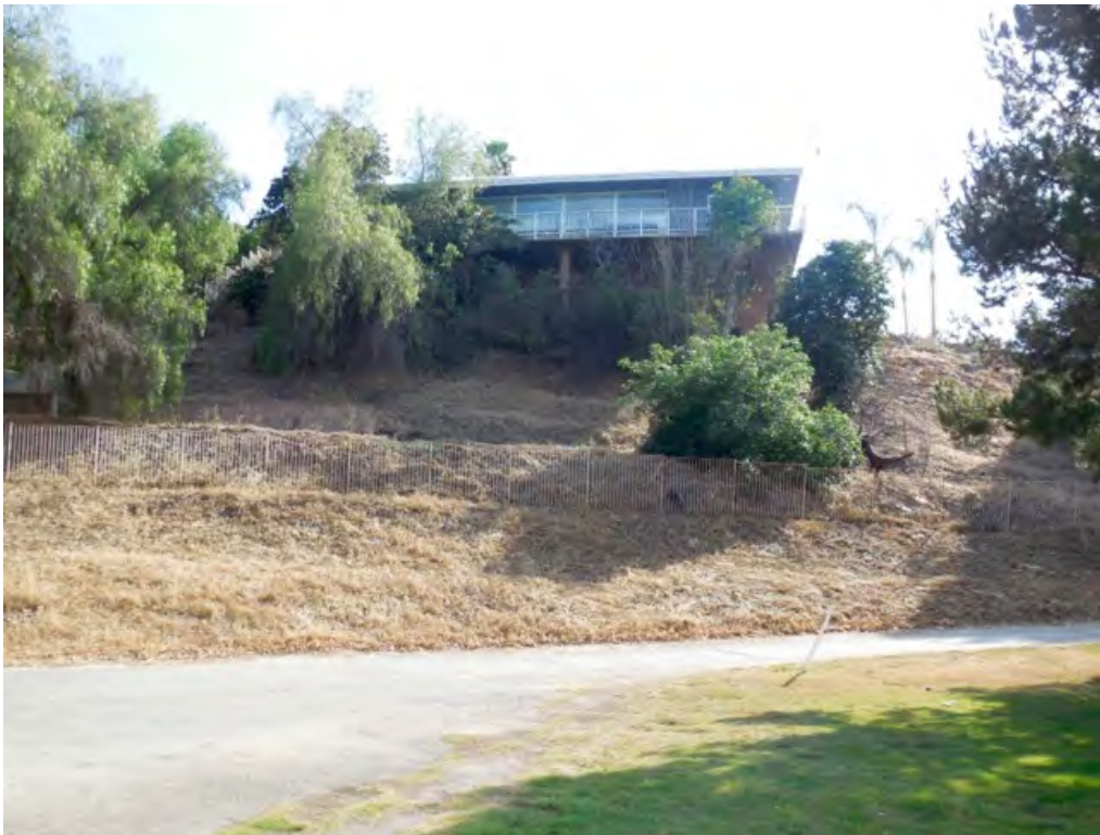
East Elevation, view looking southwest
