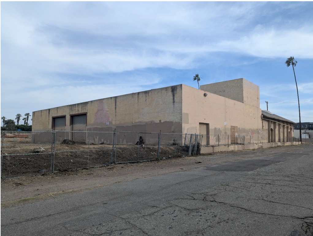
Figure 4 - Non-original addition, north and west elevations, view looking southeast
