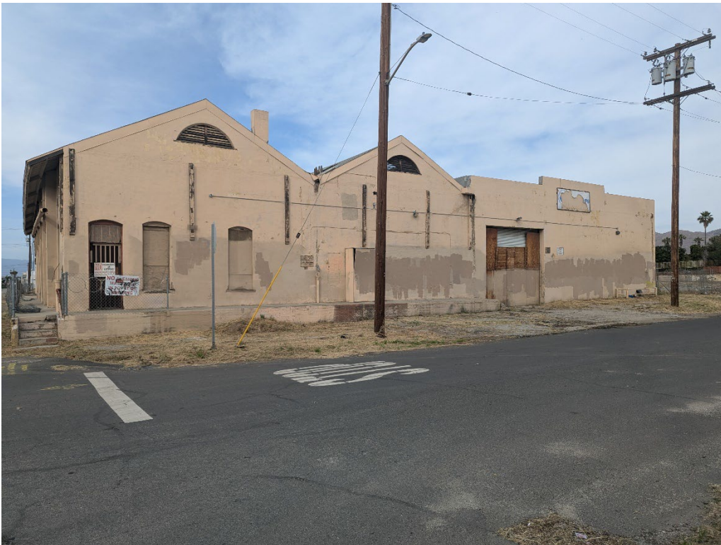
Figure 2 - South elevations, view looking north
