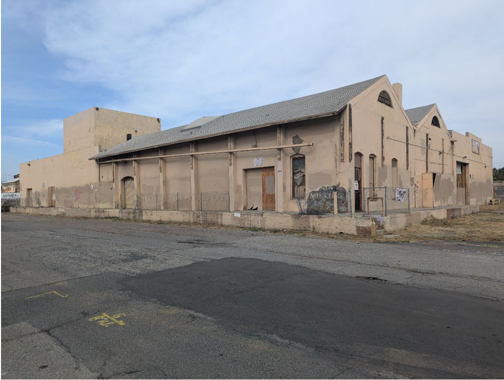
Figure 1 - West and south elevations, view looking northeast
