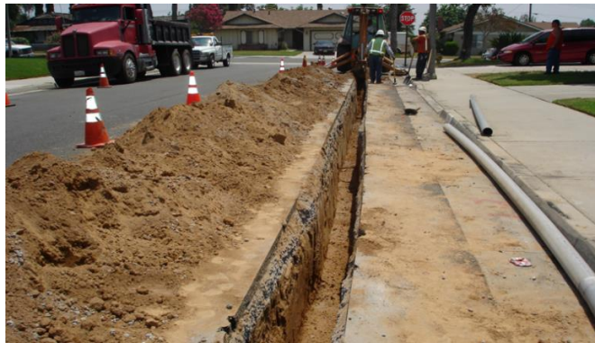
Typical Trench and Conduit Installations
