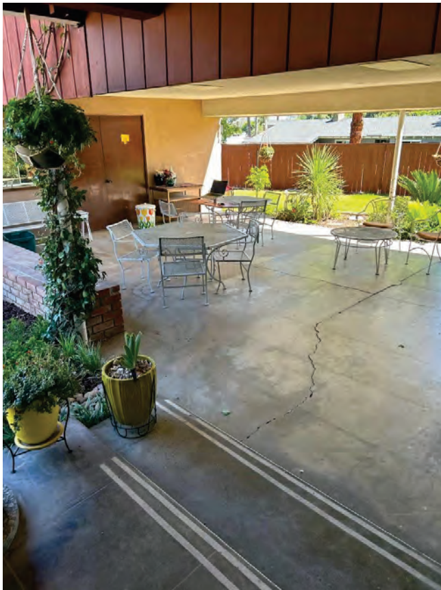
Patio highlighting indoor/outdoor living and passive cooling features.
