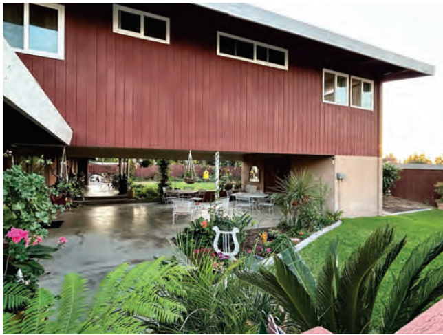
View looking from side yard: Second Story bedrooms and baths with covered patio under. Large overhanging eaves are observable on both stories.
