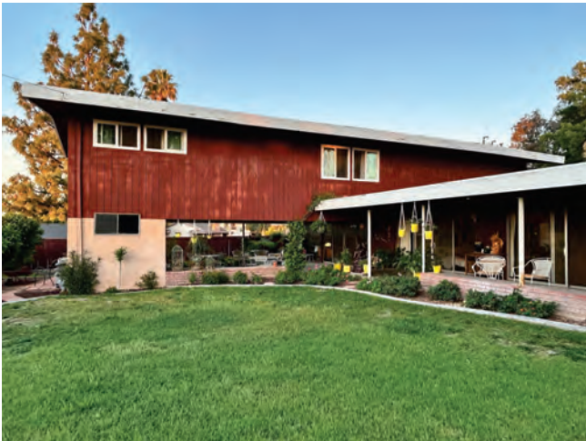
View looking from backyard: Second Story with covered patio under it and adjacent portico. Shows examples of long, horizontal massing and passive cooling features of home.
