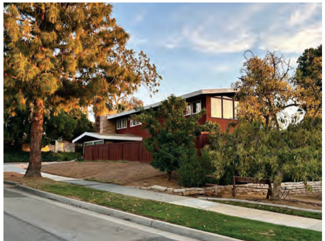
View Looking South, up Fielding: Master Suite with large original clerestory and single pane windows.
