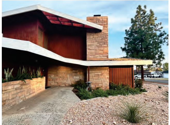
Main Entrance showing desert rock veneer chimney and planter as well as eggcrate cutout
