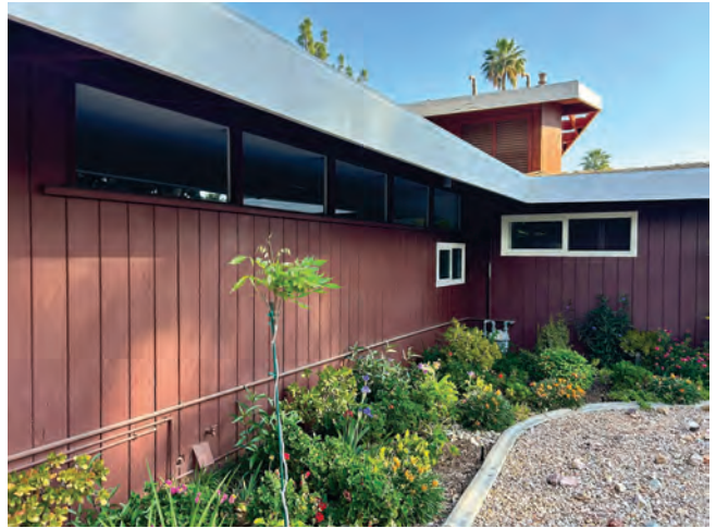
View of original kitchen clerestory windows under overhanging eaves.
