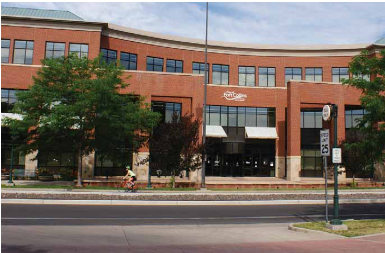
This municipal building has solar photovoltaic (PV) systems.
