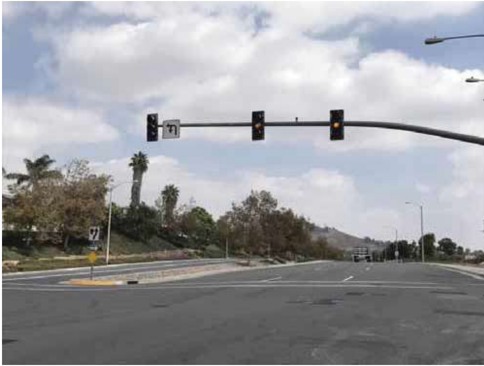
Photo 9: Residential Conflicts: Limonite Avenue.
