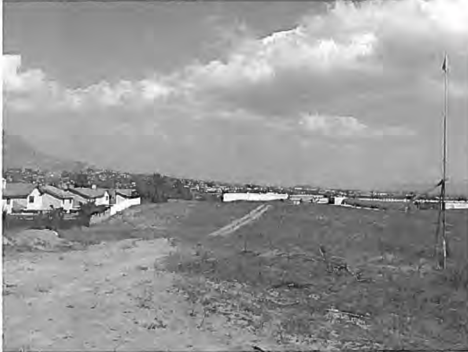
Figure 7 - A view from the East along the northern residences line. The wall is expected to extend from this location for about 850 feet about 100 feet from the residences shown on the left, clearly towering over the existing homes. Other corner flag to far away to be seen in this picture (850 feet)
