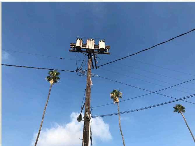
31. Pole-mounted transformers
