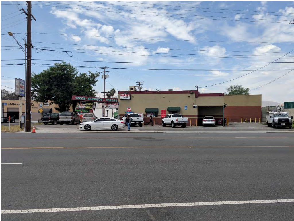
View of the site looking west.
