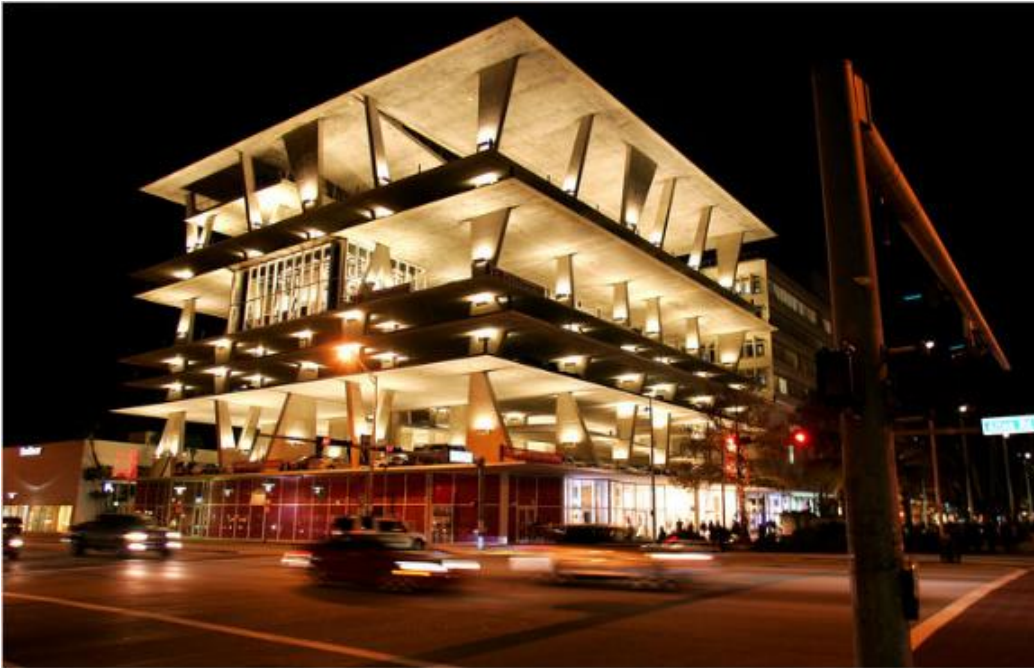
Miami Lincoln Parking Structure in Miami, Florida
