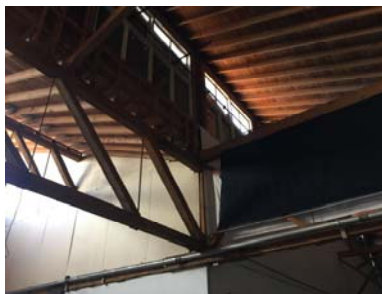
Saw-toothed roof with clerestory windows
