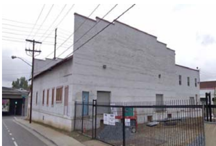
South and East elevations with example of Western False Front style stepped parapet and loading bays
