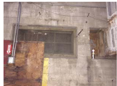
Basement ventilation windows
