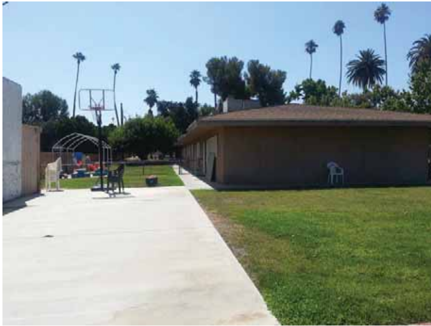
3. View of East Boundary and Northeast Building, Looking South.
