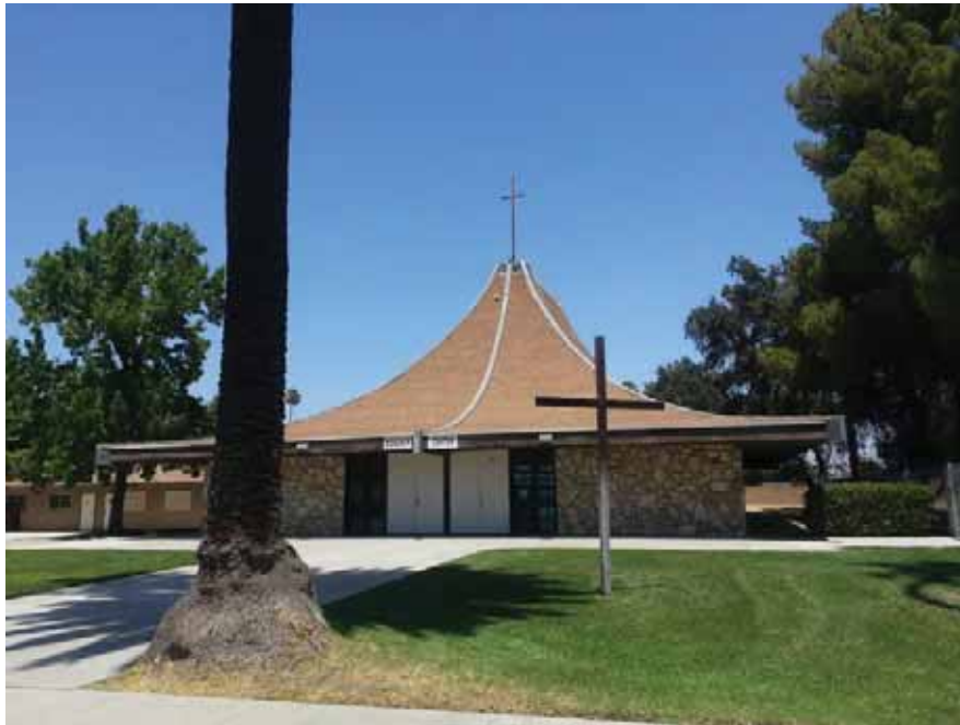
5. View of Church Building, Looking East.
