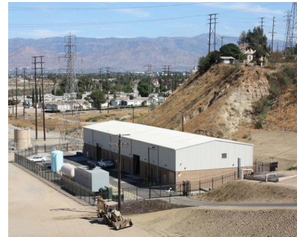
John North Water Treatment Plant
