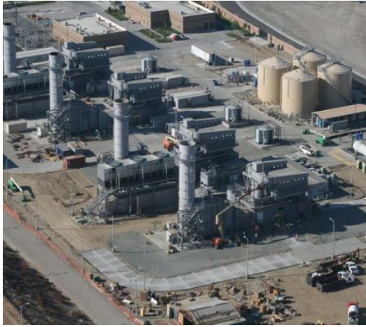
RERC Electric Generation Units
