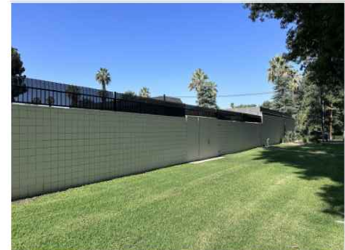
MATCH EXISTING 12' CMU WALL WITH 2' TUBE STEEL FENCE
