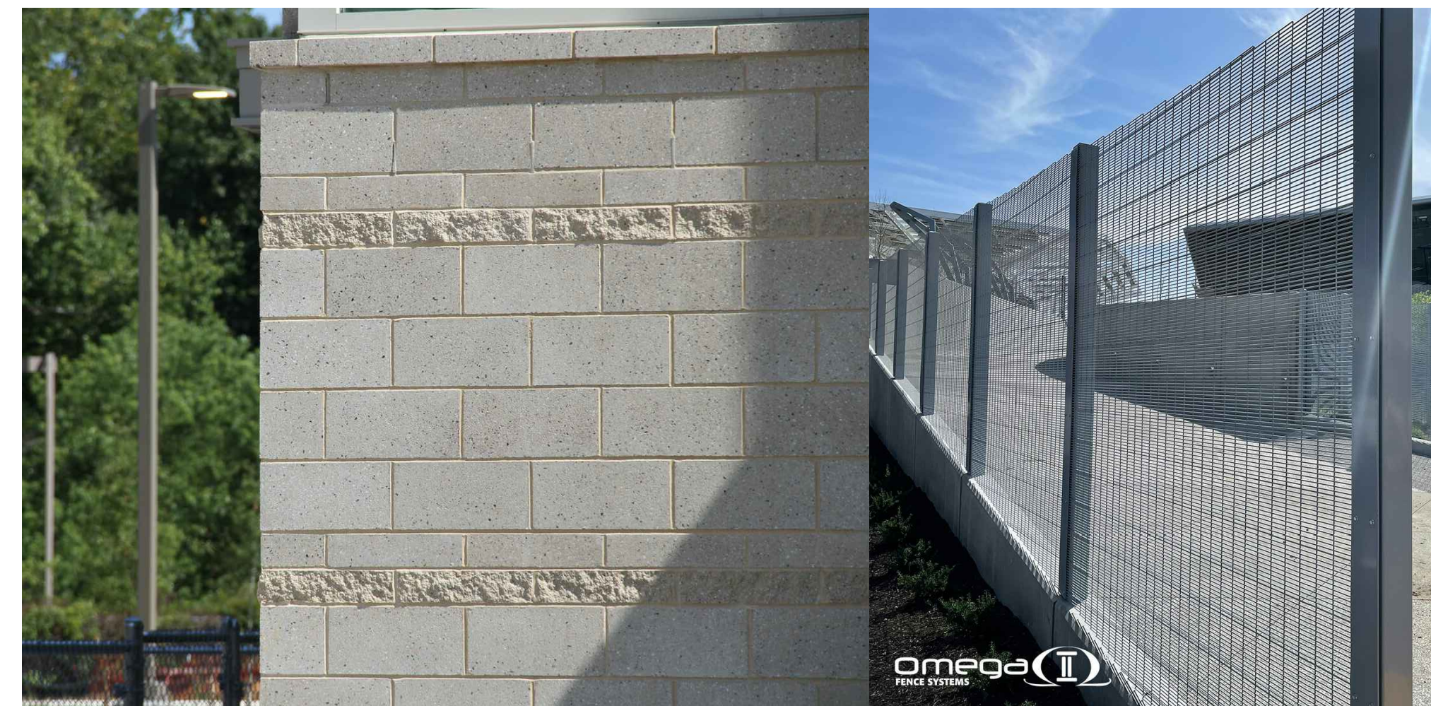
9' TALL INTERIOR CMU WALL WITH DECORATIVE BANDS WITH 5' TALL OMEGA MAX FENCE PANEL ON TOP OF WALL.
