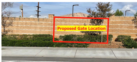
Existing Block wall at La Colina Substation
