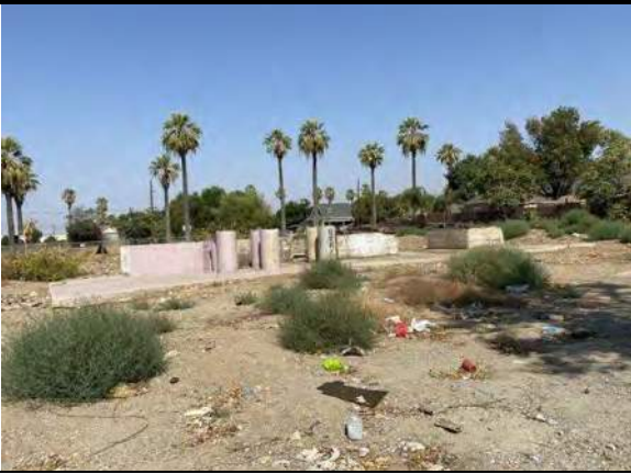
View of former concrete pads for former bailer and cranes on the 2993 6 th Street parcel
