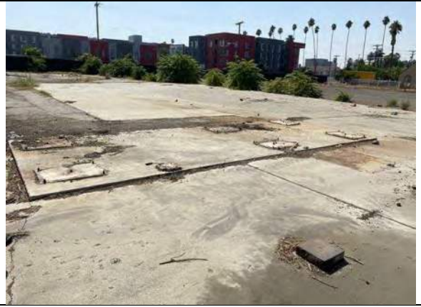
View of former building pads
