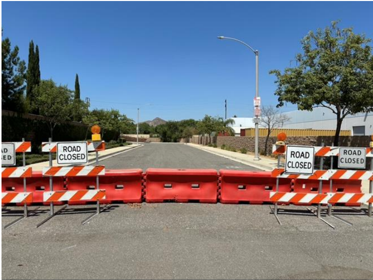
Figure 1: Photograph of interim water-filled barricade improvements.
