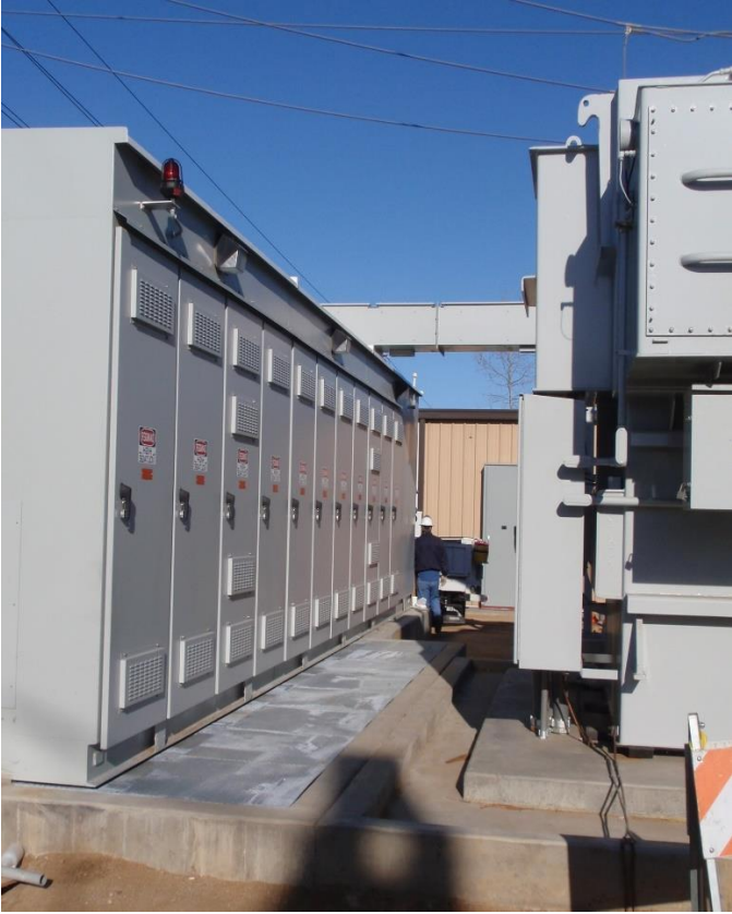
Proposed new transformer and switchgear equipment at La Colina Substation
