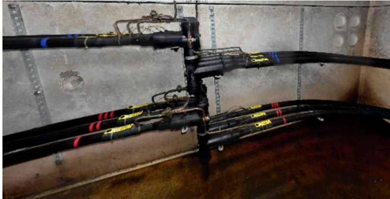
Underground Primary Feeder Cables inside the Vault
