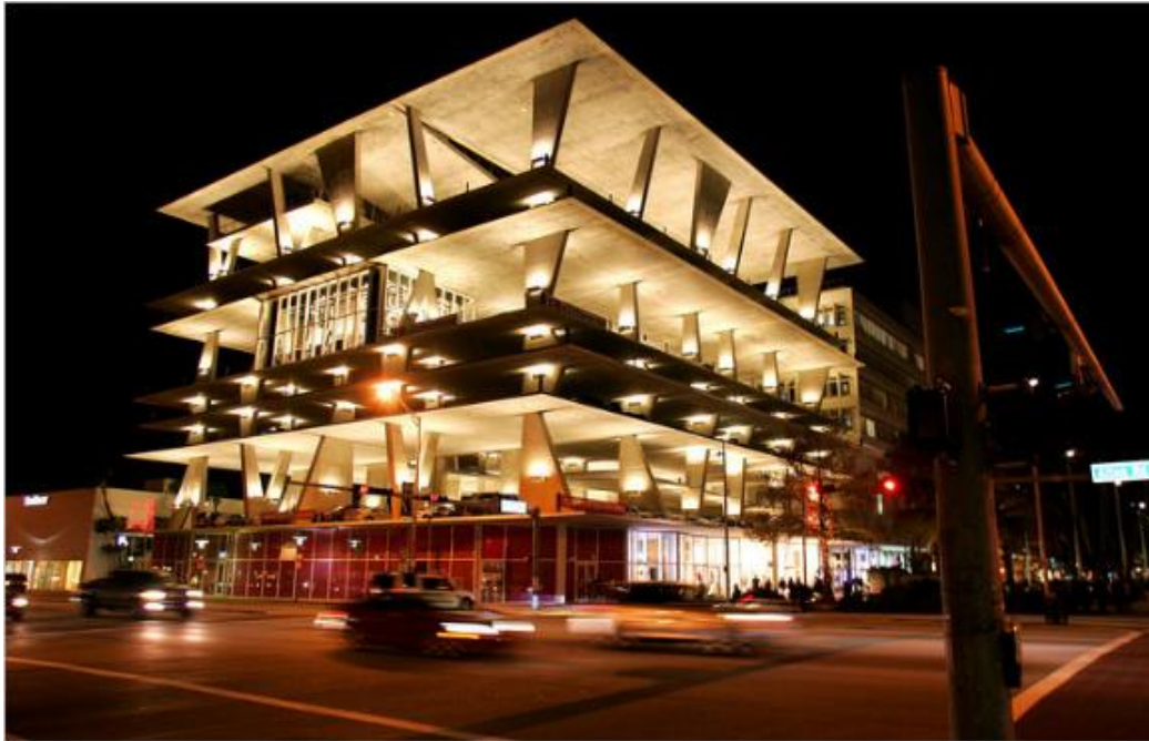
Miami Lincoln Parking Structure in Miami, Florida
