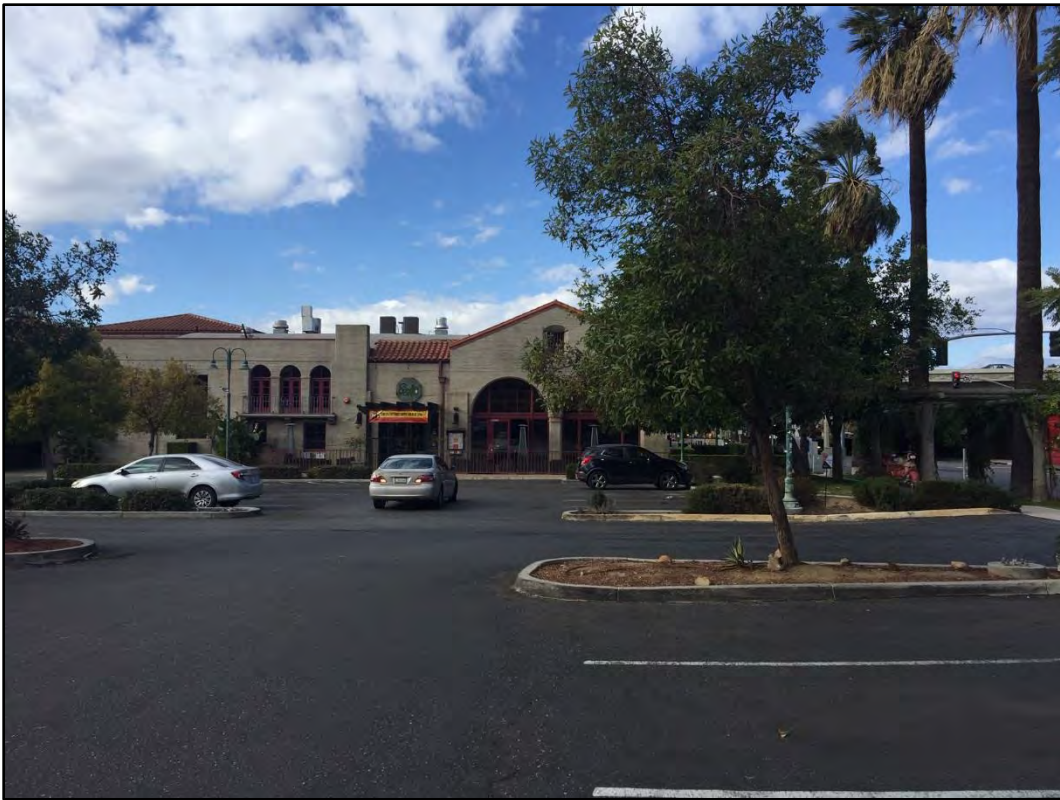
Taken from the parking lot looking west.
