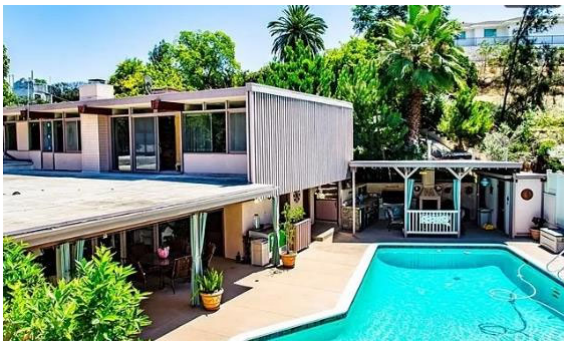
North elevation of third story & Pool Deck
