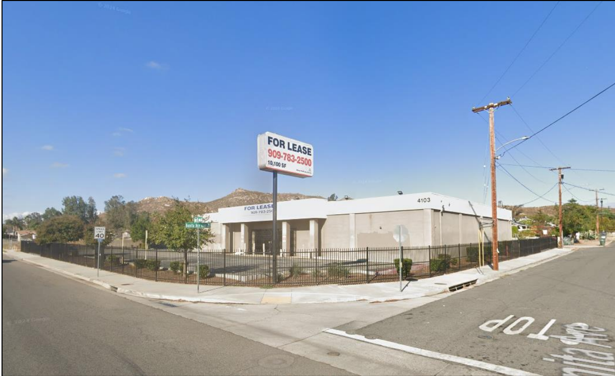
Facing northwest to the project site, from intersection of Tyler Street and Bonita Avenue
