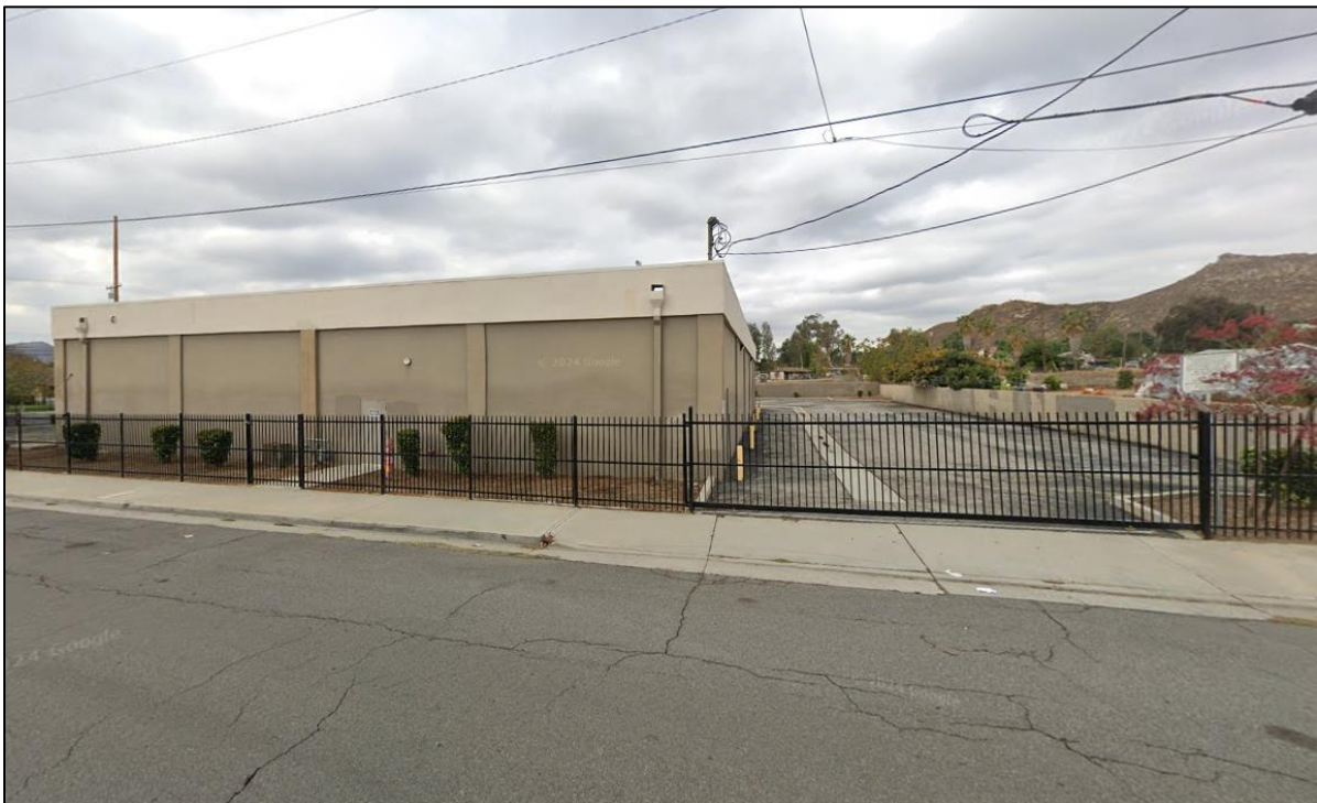
Facing west to the project site, from Bonita Avenue
