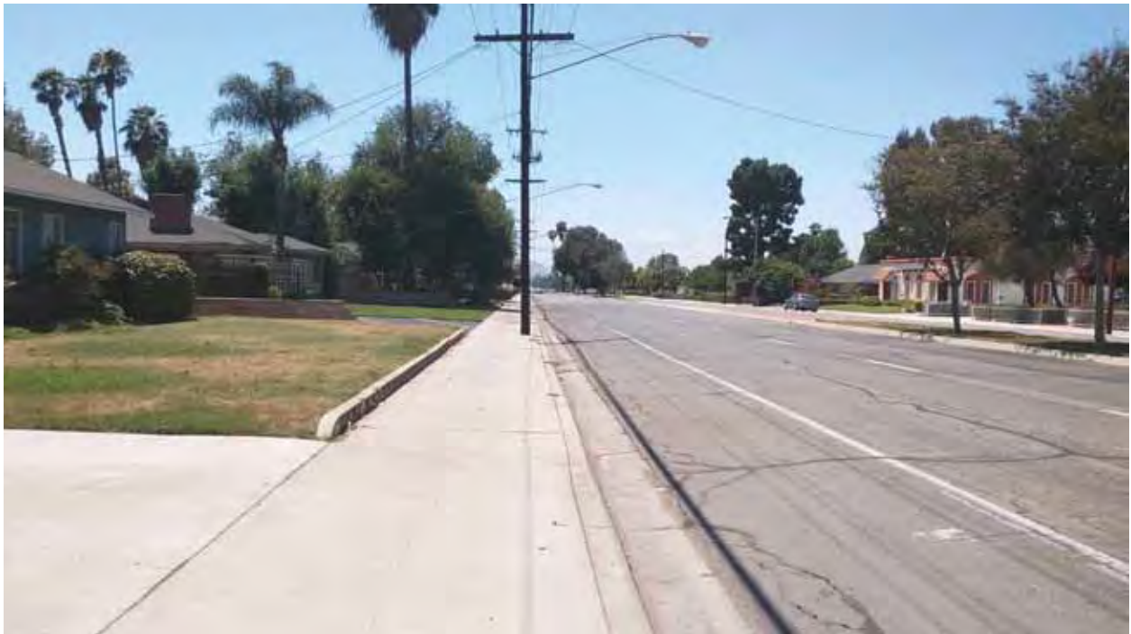
View looking west on Arlington Avenue
