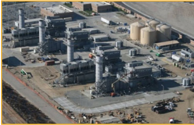
Riverside Energy Resource Center (RERC)
