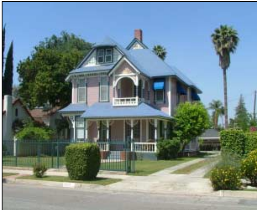
The Magee House (1888) at 4529 Sunnyside Drive
