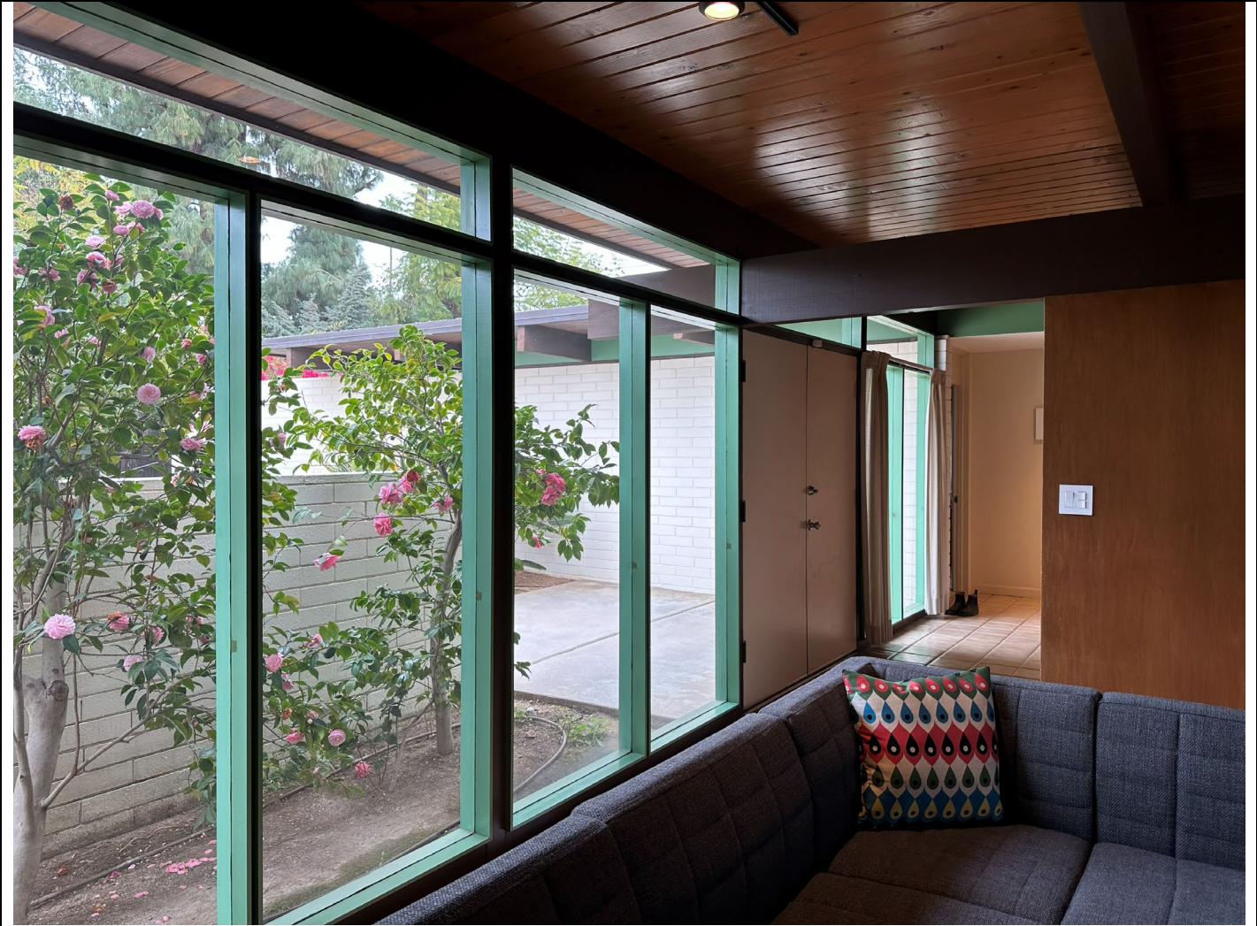
Interior view of façade fenestration and continuation of open beam and ceiling boards, view northeast
