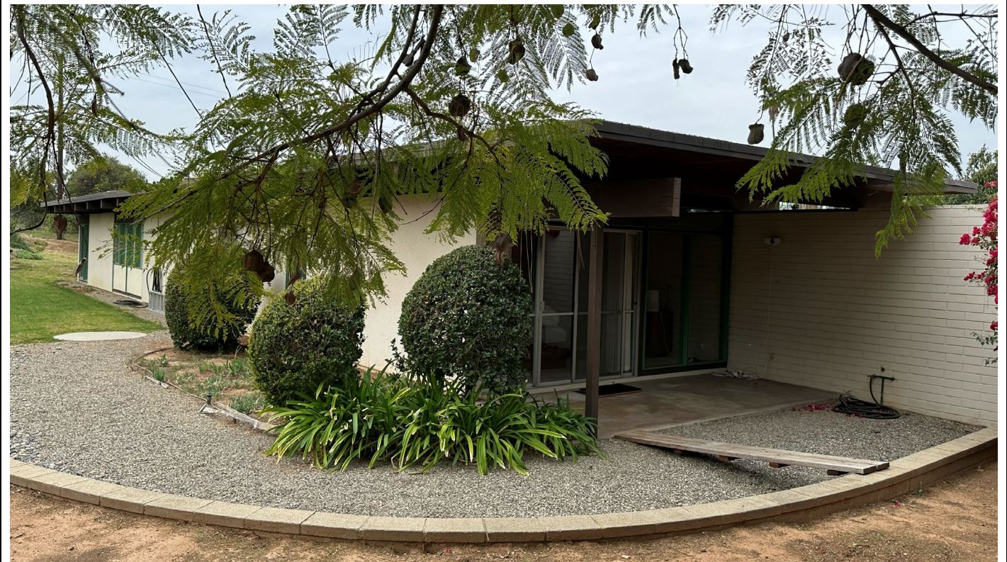
East side/rear elevation showing small patio behind secondary front elevation block wall, view southwest
