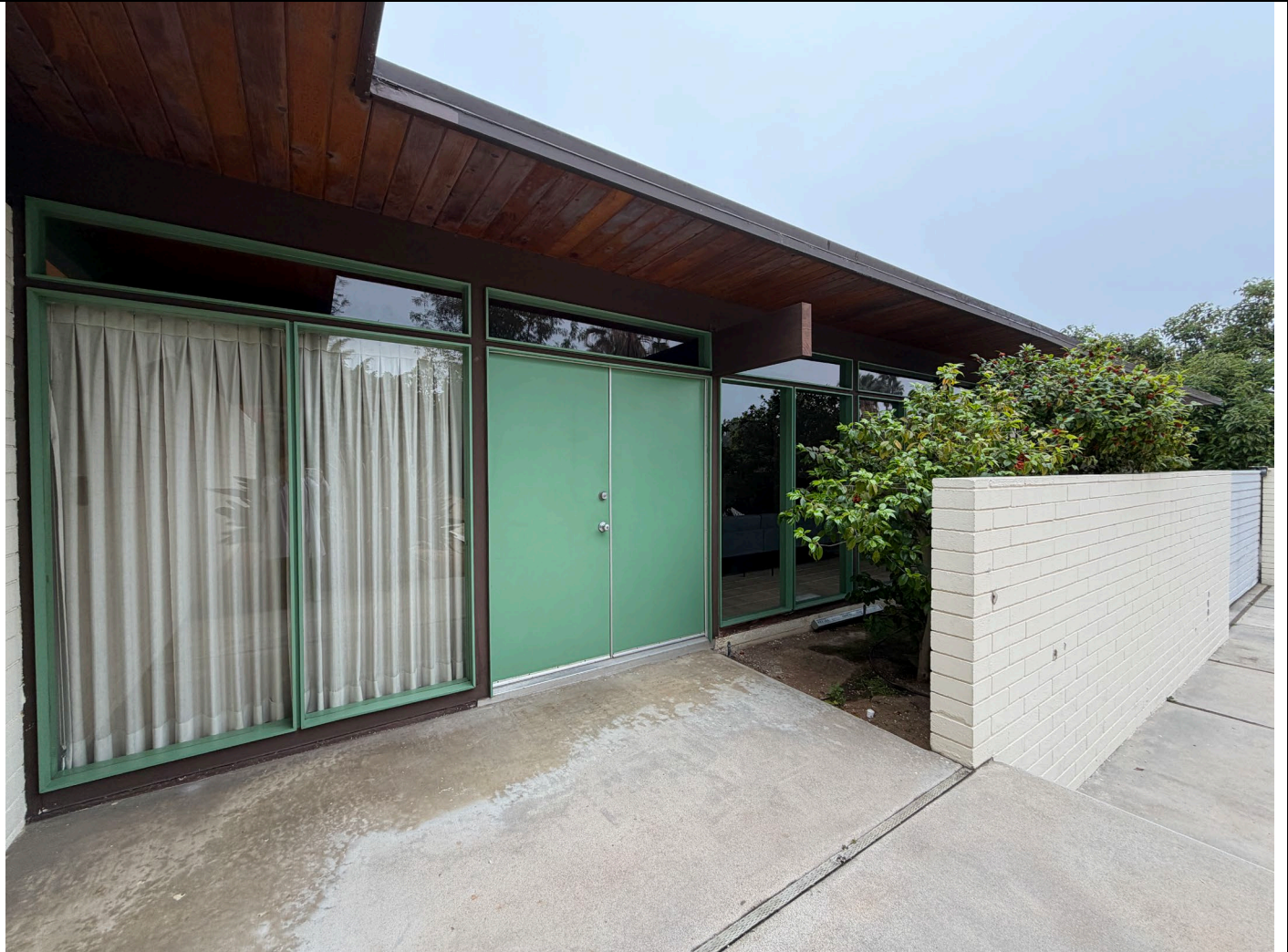
Edie façade fenestration, eave, and roof beams behind freestanding garden wall, view southwest
