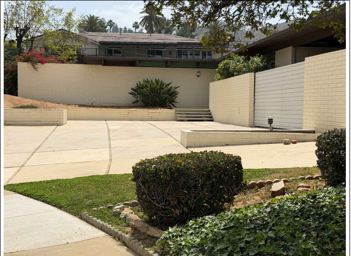
Edie façade, secondary front elevation, and driveway, view east/southeast
