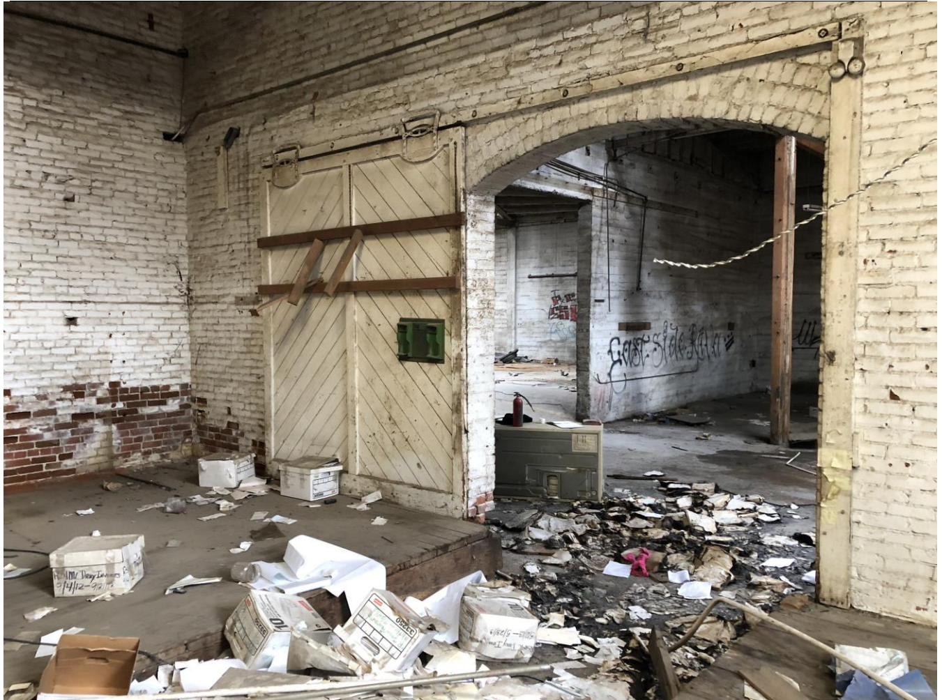
Barley Mills Building Interior: Source G T Louden AIA Photography, February 2022; Figure # D-15 View to east of original triple wythe segmented brick arch opening in original east exterior façade. View through opening is of the concrete walls structure of the later 1930 additions.
