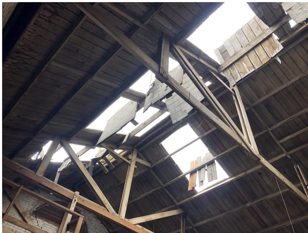
Barley Mills Building Interior: Source G T Loudon AIA Photography, February 2022; View of wood roof framing, board finish at the joists; the south wall brick façade and the half circular vent; the roof openings for skylights are not original and are not proposed to be restored. Figure # D-18
