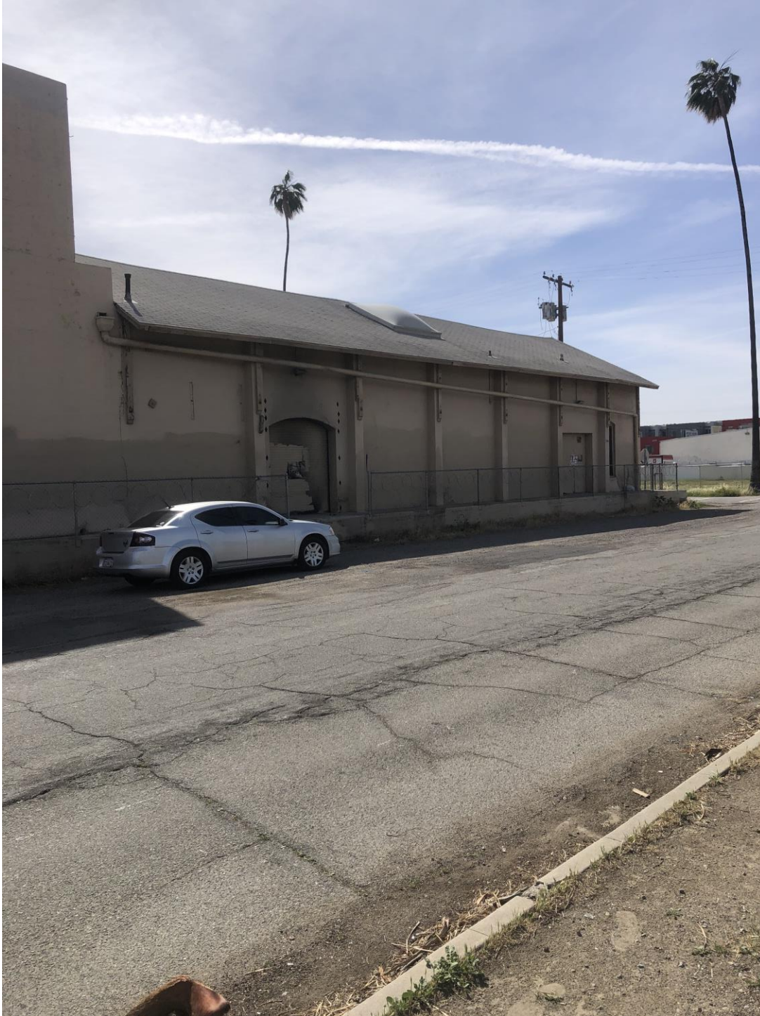
Barley Mills Building Exterior: Source G T Loudon AIA Photography, March 2022; Overview of west façade; the taller mass at the left side is part of the 1930 era addition; skylights are not original and are not proposed to be restored. Figure # D-19
