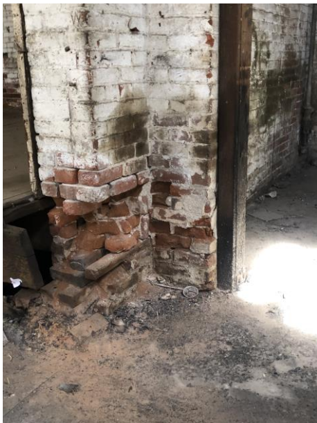
Barley Mills Building Interior: Source G T Loudon AIA Photography, March 2022; Interior view of south east façade, near the corner; note the brick masonry foundations have failed at the original west façade opening at the former exterior doorway jamb; Figure # D-21.
