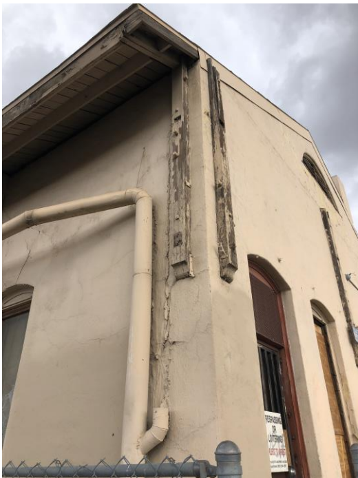
Barley Mills Building: Source G T Loudon AIA Photography, February 2022 ; Existing Conditions at corner, including wood brackets for attachment of non-extant canopies south façade door and window rough openings; Figure # D-10
