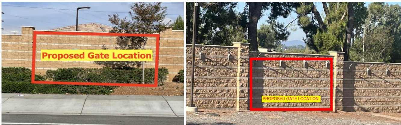
Existing conditions outside and inside La Colina substation
