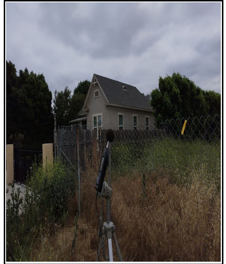
STNM4 looking S towards closest residence 3008 4th Street, Riverside.
