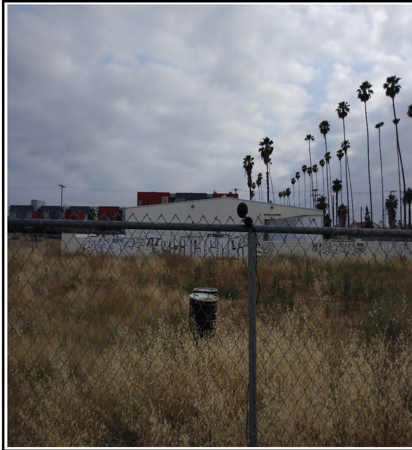
LTNM1 looking SW across site area towards building 3093 Mission Inn Avenue, Riverside.
