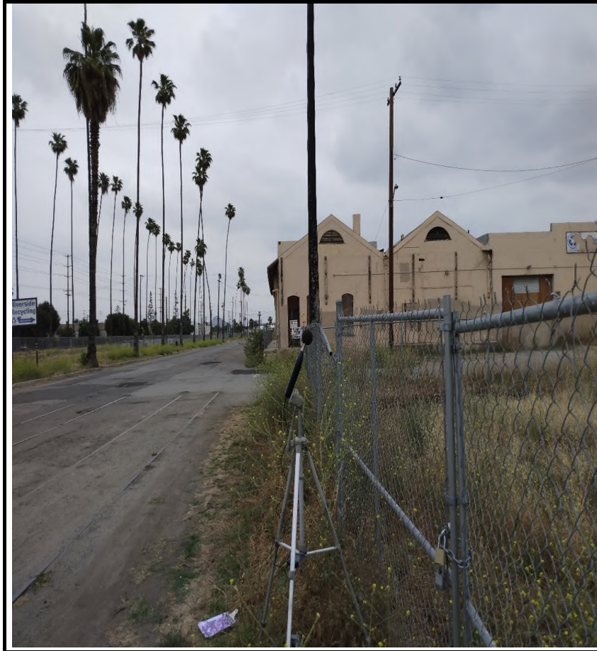
STNM5 looking NE down Commerce Street towards 6th Street intersection (~70'). Unoccupied building 3596 Commerce Street.
