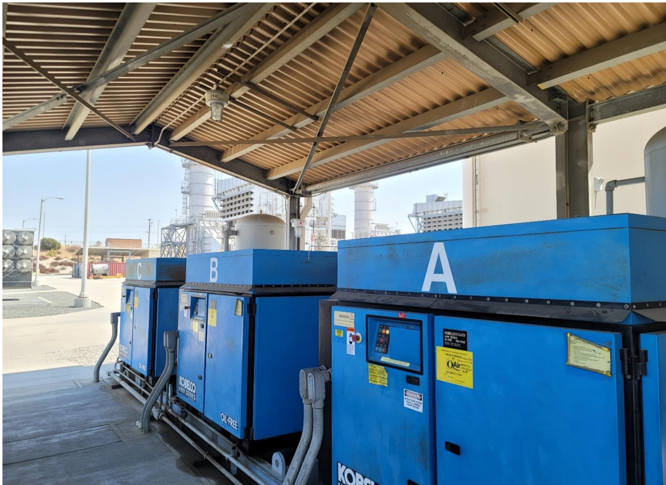
Figure 1: Three Air Compressors for RERC 1&2
