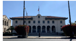
Maintaining 4 historic sites (7 sites total)
