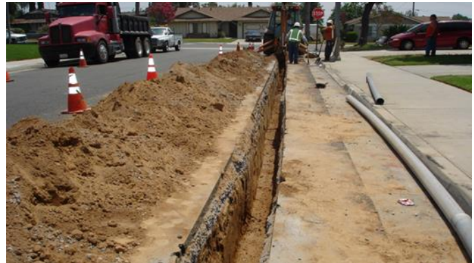
New trench and conduit installations
