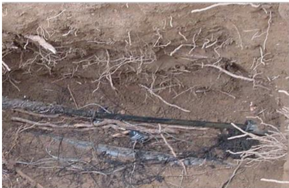
Aged Infrastructure: Cable-in-Conduit System
