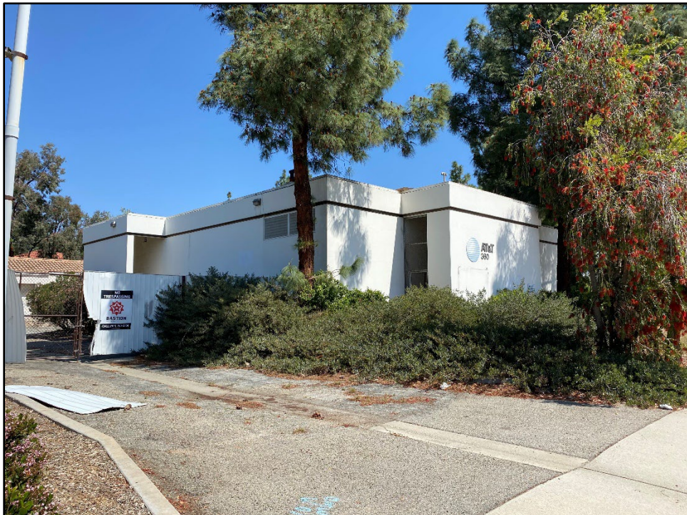
Looking east at the project site, from Alessandro Boulevard.
