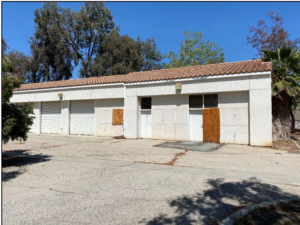
Existing building on site, along the north property line.
