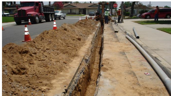
Trench and Conduit Installation
