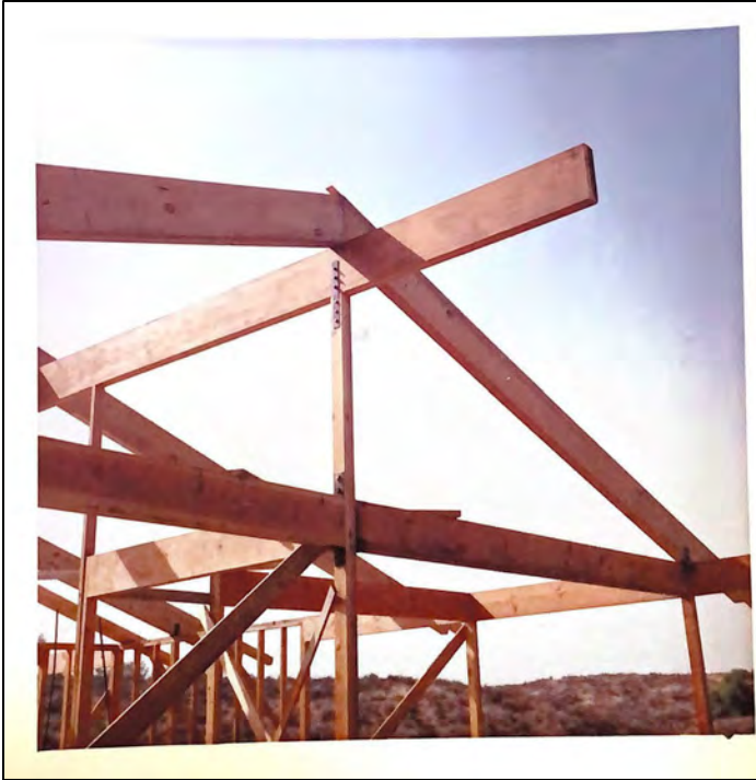
Polaroid 3 (front/back) To give you an idea of the post and beam construction. Beams are 4 inches by 14 inches and 16 feet long to 20 feet long.
