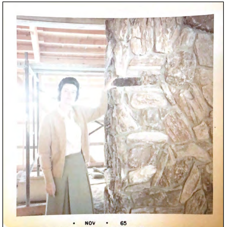
Polaroid 3 (front/back) To give you an idea of the post and beam construction. Beams are 4 inches by 14 inches and 16 feet long to 20 feet long.
