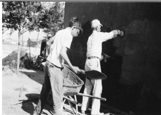
Figure 26: 1952 image of a plasterer applying stucco to a former barracks building (Frank Teurlay)
